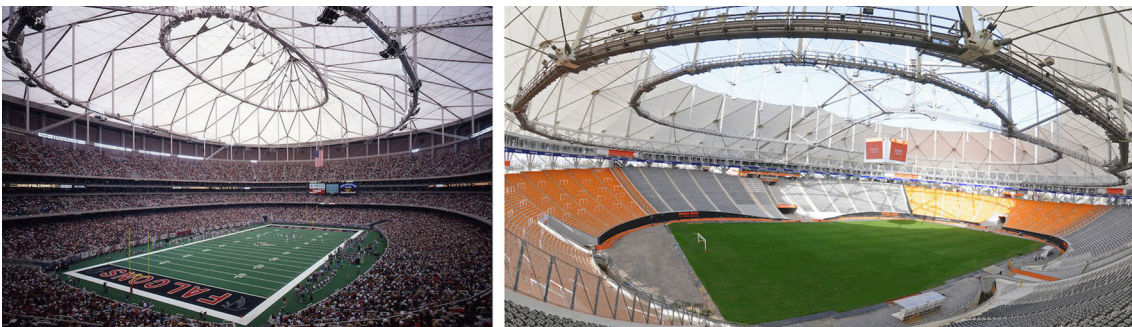
Fig. 9 The Georgia Dome (left) and the La Plata Stadium . (Left image from https://www.birdair.com/birdair-portfolio/georgia-dome/ ; right image from https://www.stadiumguide.com/ciudaddeplata/ )
