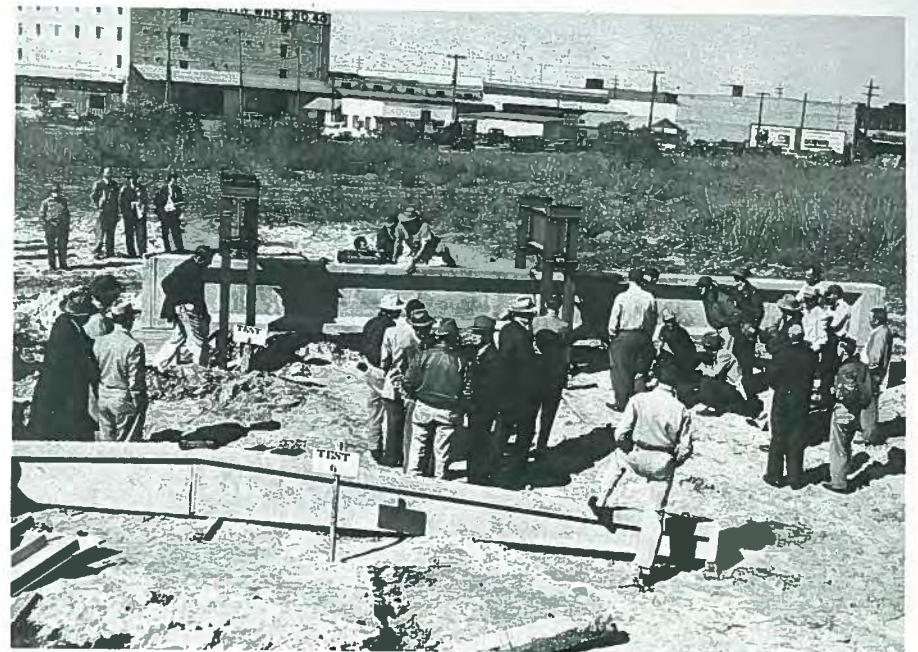
Fig. 26. Demonstration test of prestressed I-beam at Cone Brothers Construction Co., Tampa, Florida. In foreground is a variable depth tee-joint. Courtesy: Paul Zia.
