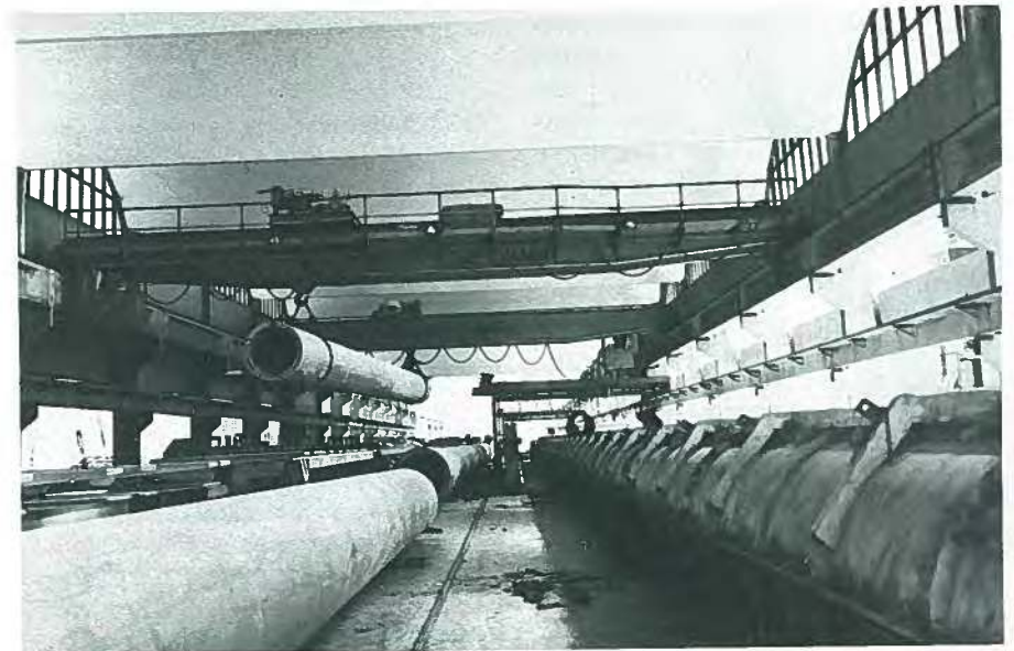
Fig. 84. Freshly cast prestressed hollow cylinder piles.
