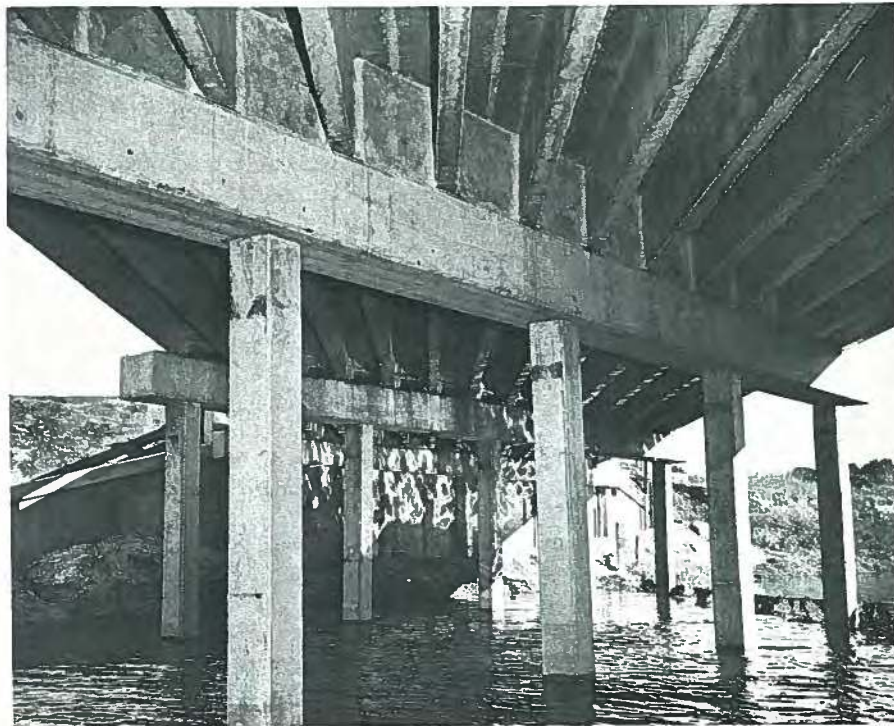
Fig. 16. Underside of precast prestressed county bridge in Sarasota, Florida. Courtesy: Paul Zia.
