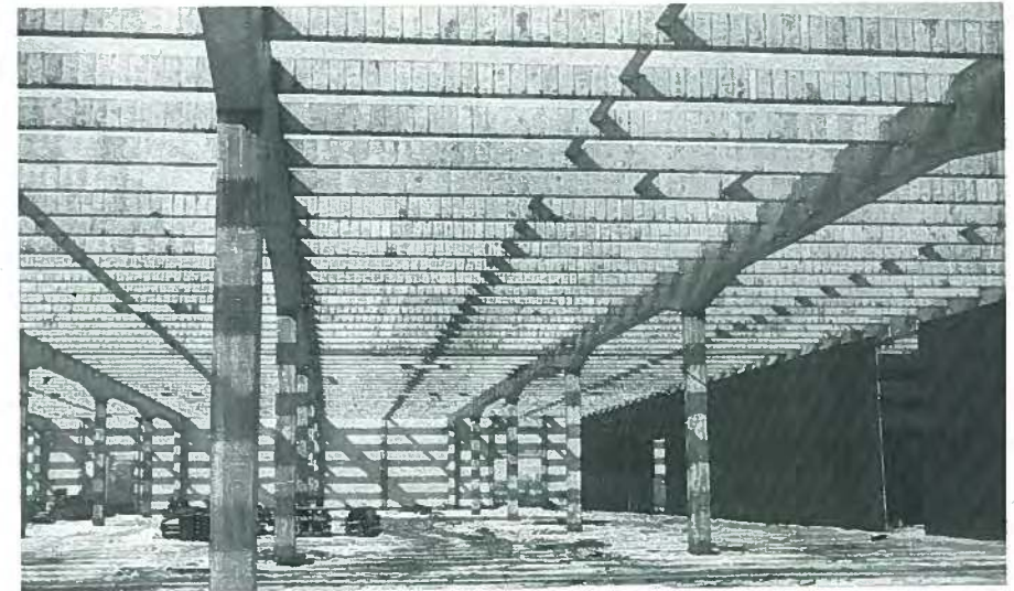
Fig. 14. Prestressed block joist on 800,000 sq ft (74,300 m 2 ) warehouse for Wilkins Air Force Depot.
