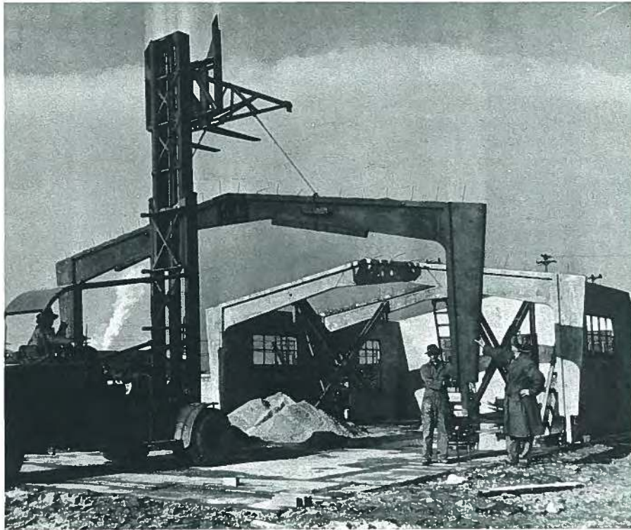
Fig. 43. Erection of Concrete Engineering Company shop building (1951).
