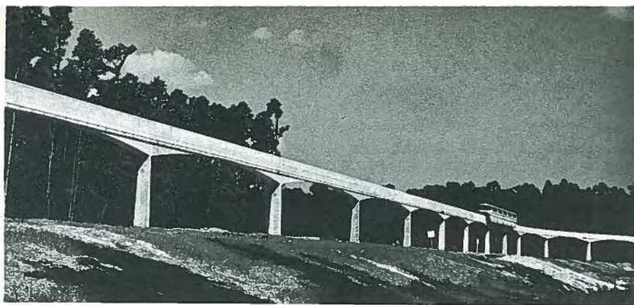
Fig. 89. The Walt Disney World monorail guideway, near Orlando, Florida, is elevated except for a few sections placed at-grade in the station areas.
