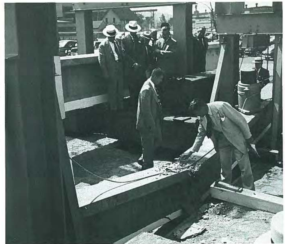
Fig. 41. After the dust settled, the author (center) and Al Waidelich inspect the fracture zone of 40-ft (12.2 m) test girder (P-40). The sudden uncontrolled failure dramatically persuaded the author to provide fully bonded tendons in all subsequent prestressed concrete construction.
