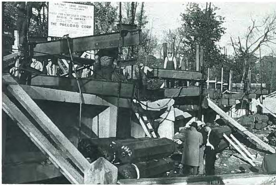
Fig. 11. General view immediately after destruction of Walnut Lane test girder. Failure occurred at 3:00 p.m., October 27, 1949.
