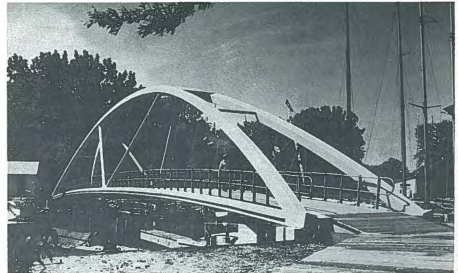
Fig. 14. Prestressed concrete footbridge for the Royal Canadian Yacht Club of Toronto, designed by L. G. Cazaly.
