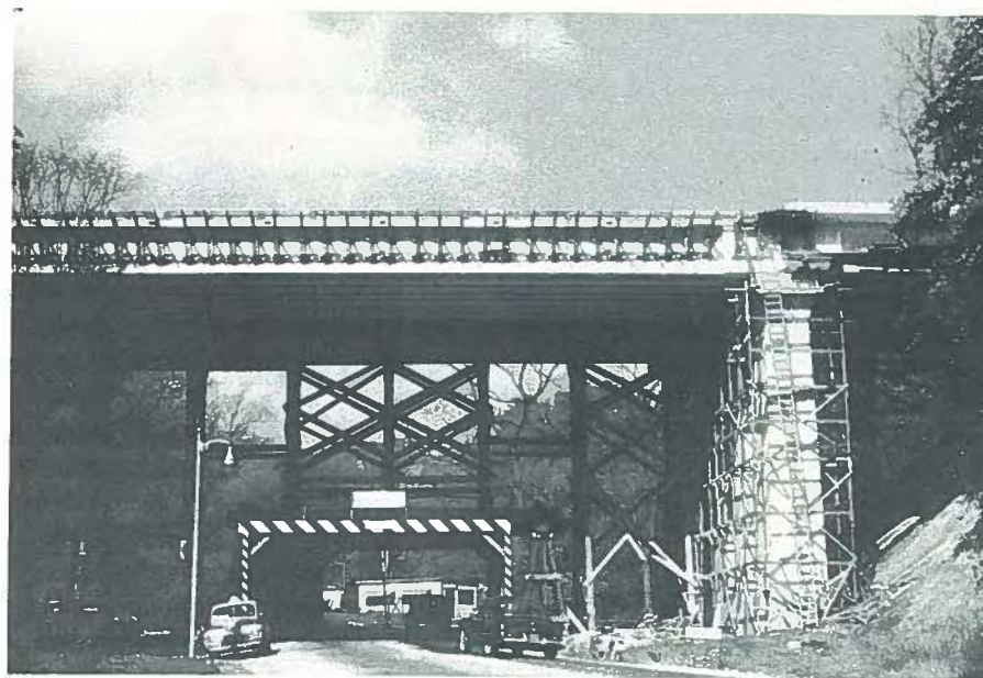
Fig. 1. The Walnut Lane Bridge under construction in 1950. Photograph shows brackets in place for formwork for sidewalk at south fascia girder.
