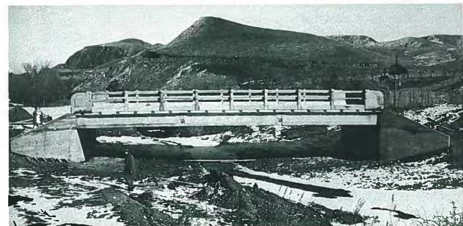
Fig. 5. The Ross Creek Bridge at Medicine Hat, Alberta, was the province's first prestressed concrete bridge (1953).
