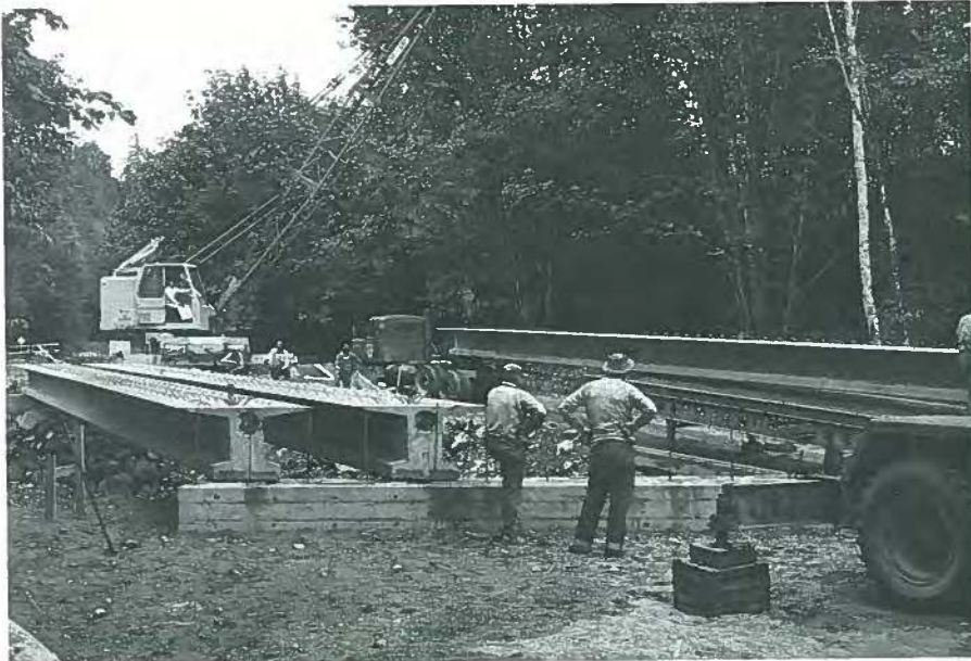
Fig. 81. Bulb T-beams being placed at erection site.
