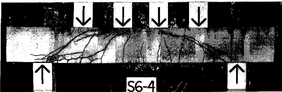
Figure B.68 Crack Pattern of the Back Face of Beam S6-4
