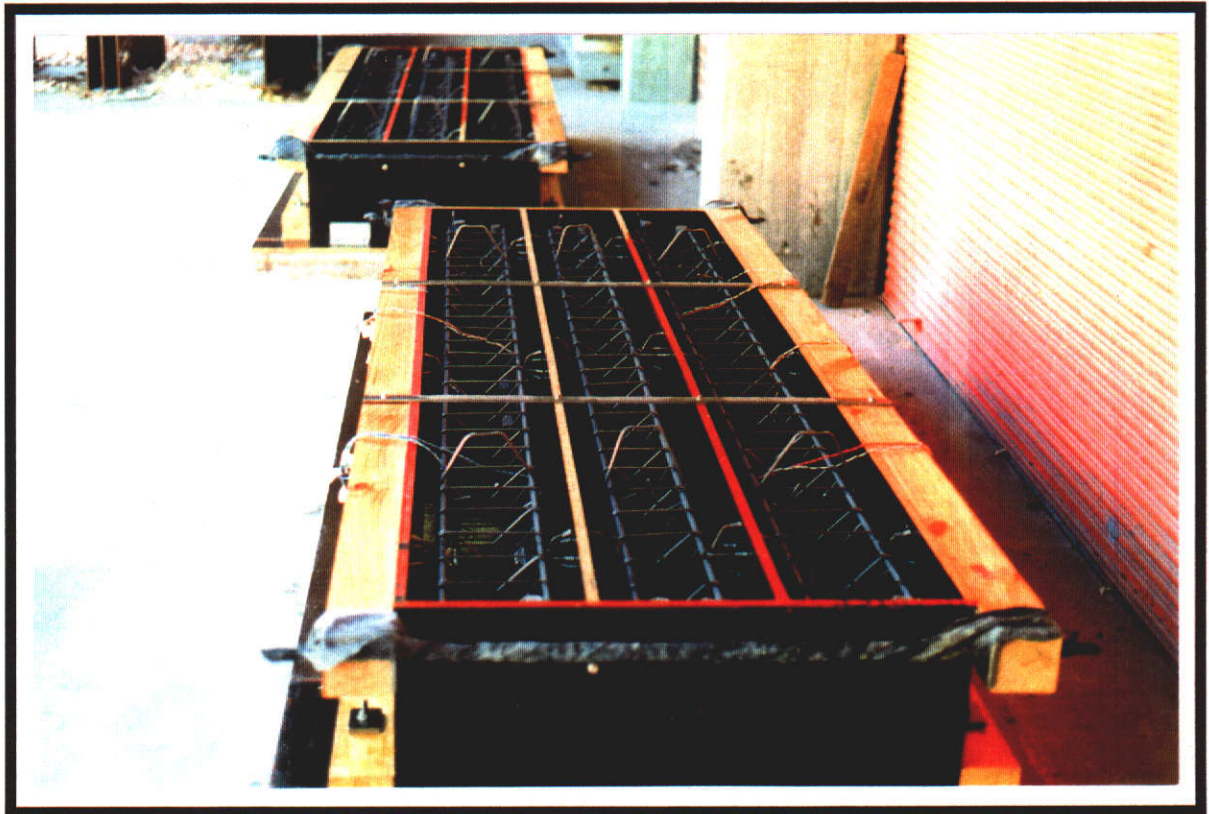
Figure 4.7 Reinforcement Cage in Timber Moulds
