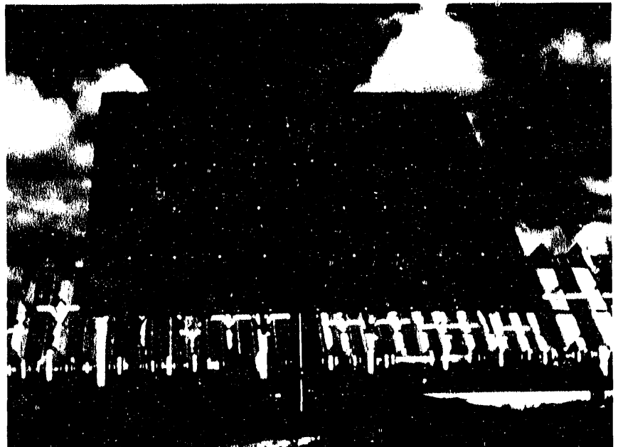
For large-scale applications, like this 6.5-MW photovoltaic system, designers prefer solar radiation data that are accurate to within 5% so they can make sound assumptions concerning system output, performance, and economics. (Photo courtesy of Siemens Solar Industries.)
