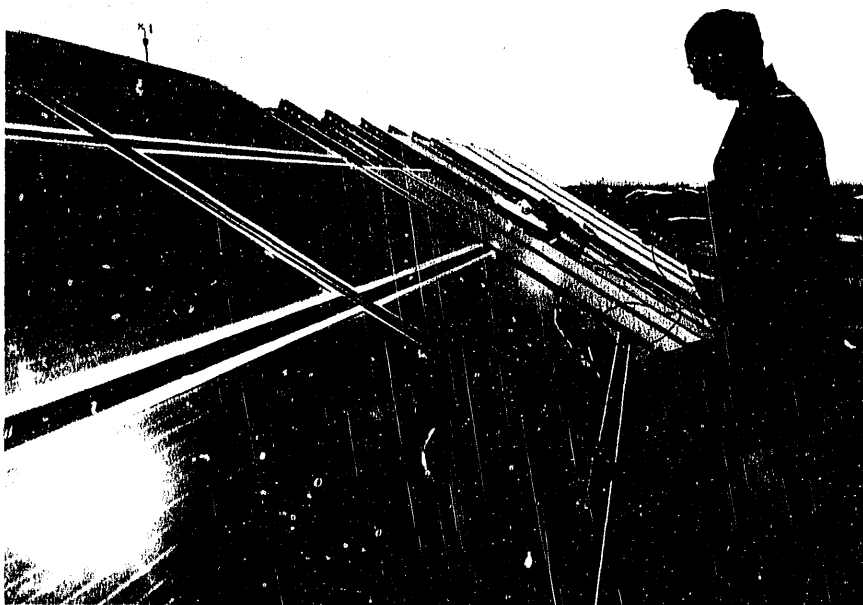
Concentrator collectors (top) use direct beam solar radiation; flat-plate collectors (bottom) use direct beam radiation, diffuse (sky) radiation, and ground-reflected radiation.
