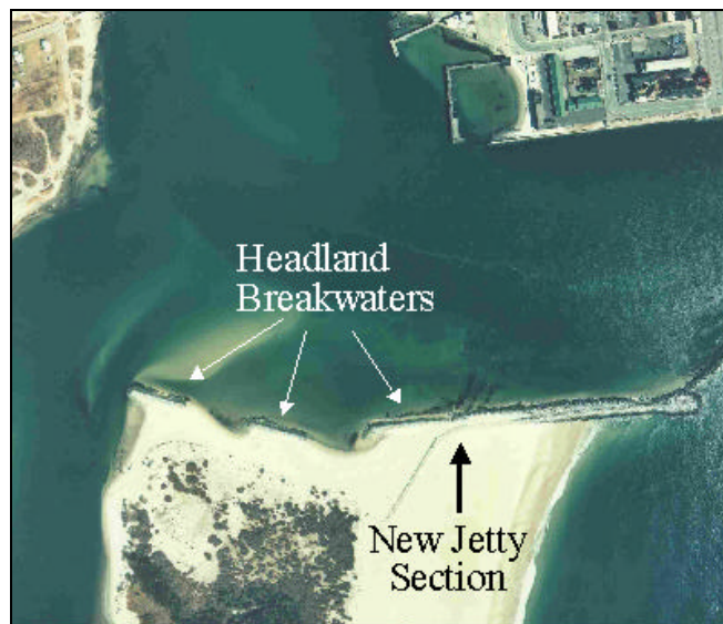
Figure 4c. Ocean City Inlet, Maryland post-project (21 Feb 1990)
