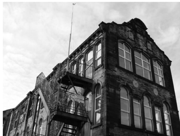
Fig. 1 Photograph of A-Block, St. Lukes Hospital, Bradford, UK
