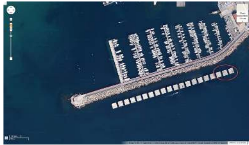
Fig. 7: Experiments scenario. Harbor of Sant Feliu de Guíxols in Catalonia, Spain, where a breakwater structure composed of concrete blocks is demarcated.
