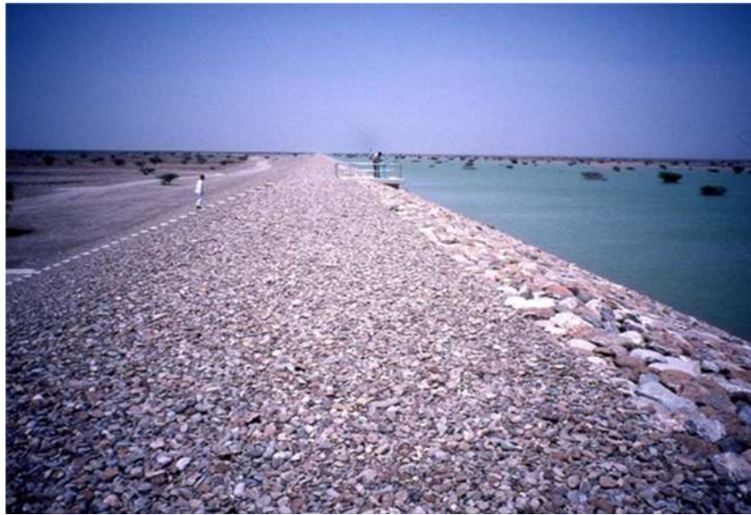
Fig. 6 Ahin recharge dam on the Batinah Plain, Oman, constructed in 1994, is a large dam (crest length 5,640 m, crest height 8 m) with a detention capacity of 6.8 Mm 3 . This is one of the 43 recharge dams, with an aggregated capacity of 95 Mm 3 constructed in Oman during the period 1985–2011 (Oman MRMWR 2012). Their purpose is to enhance aquifer recharge primarily to support irrigation; and also to protect the
