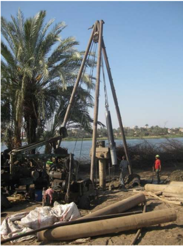
Fig. 7 Drilling of riverbank filtration wells at the Nile River, Luxor, Egypt, March 2018. Seasonal low river water level, frequent spills of oil and other pollutants and high turbidity during high flow cause problems in surface-water abstraction and subsequent treatment. A short distance between the abstraction wells and the river bank is sufficient to remove particles, to buffer spills and to ensure a high portion of bank filtrate and a low portion of manganese-rich land-side groundwater (Photograph courtesy of T. Grischek, University of Applied Sciences Dresden, HTWD)
