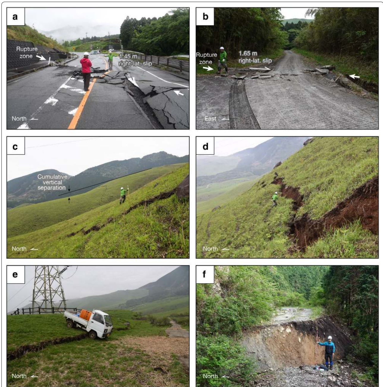
Fig. 4 Photographs of features of the 2016 Kumamoto earthquake surface rupture. a Displaced centerline of the paved road next to the Okiribata dam. Arrows point along fault trace. b Pure right-lateral slip of the concrete road. Arrows point along fault trace. c Normal fault scarp cut a grass slope in a ranch. Coseismic vertical separation at the site is ~1 m, but the cumulative topographic offset is evident. d Free face of the unconsolidated soil and volcanic ash unit on a normal fault scarp in the grass slope. e Uphill-facing normal fault scarp on a grass slope. It is interpreted as an antithetic fault. f Maximum ~2.0-m vertical separation of a forestry road
