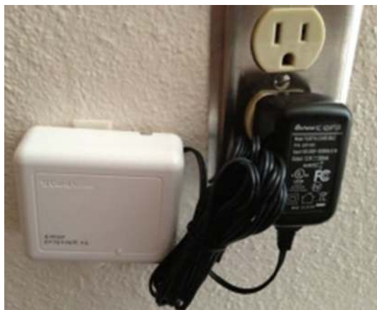
Fig. 2 An illustration of an installed relay on the wall
