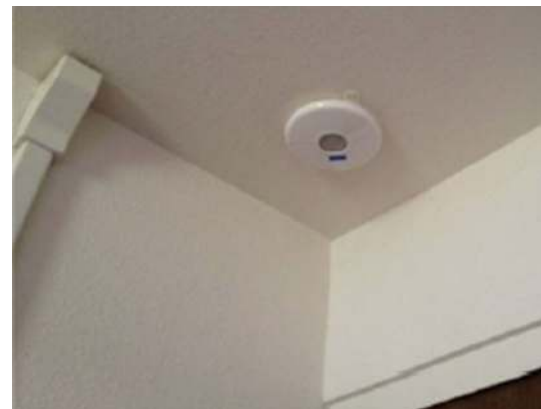
Fig. 3 An illustration of correct way to install a motion sensor
