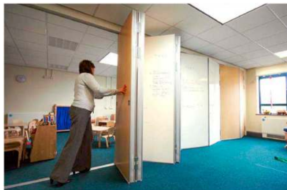
Figure 2. Example of removable partition wall (Dividers, 2014).
