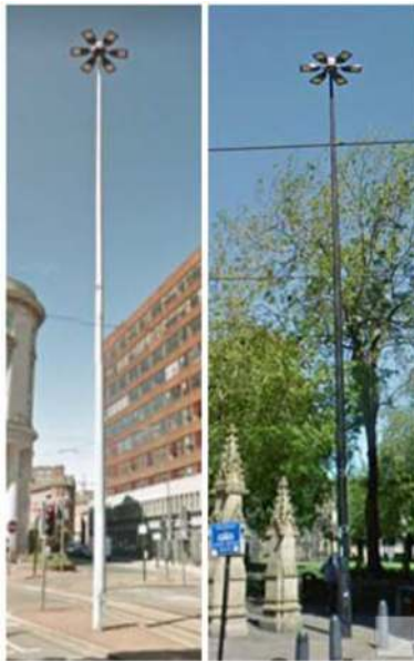
Fig. 13 Church Street streetlights
