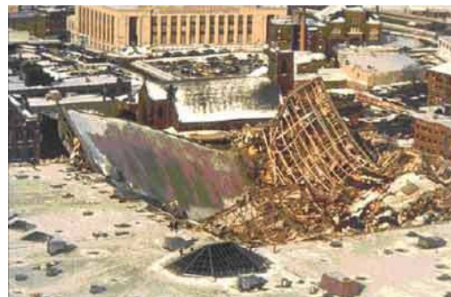
Figure 2. Hartford arena roof collapse. *
