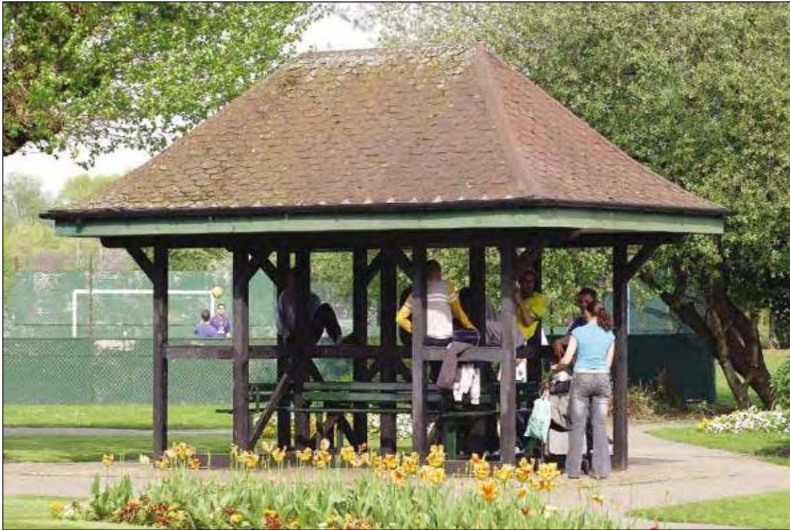
Vale Park: covered benches
