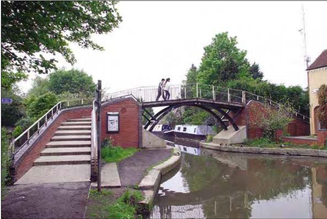
Canal: towpath and bridge
