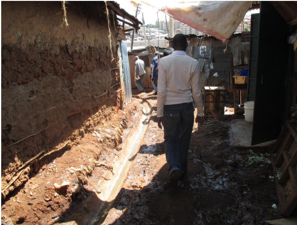
Plate 4. A typical drain and housing structure in Kibera. Photo by authors during survey.
