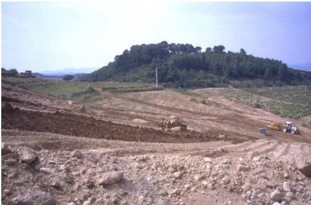
Figure 2. b) Land levelling in the Penedès region to adapt vineyard to mechanization. 22x14mm (600 x 600 DPI)
