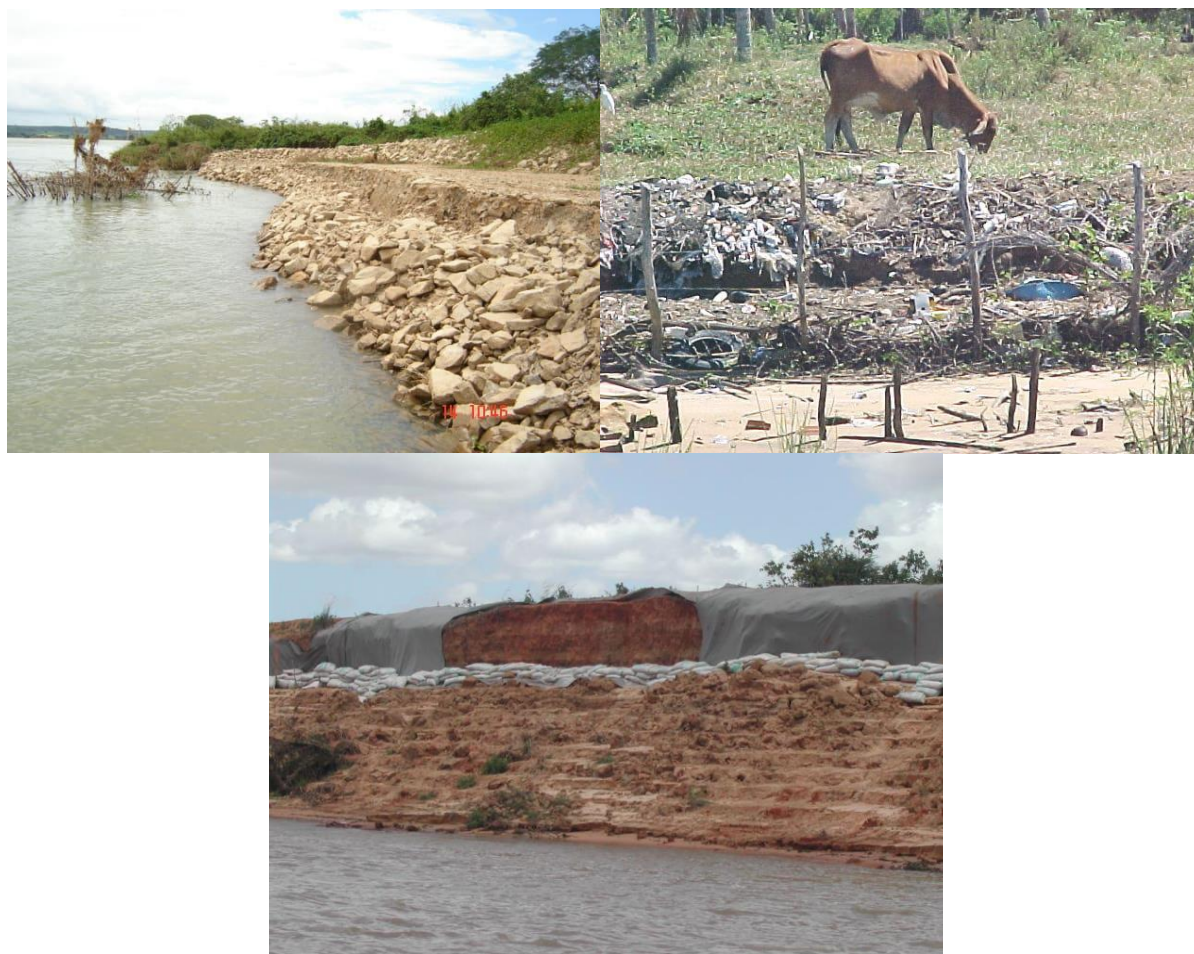
Figure 5. Riprap and other erosion-control methods used by the riverine population.
