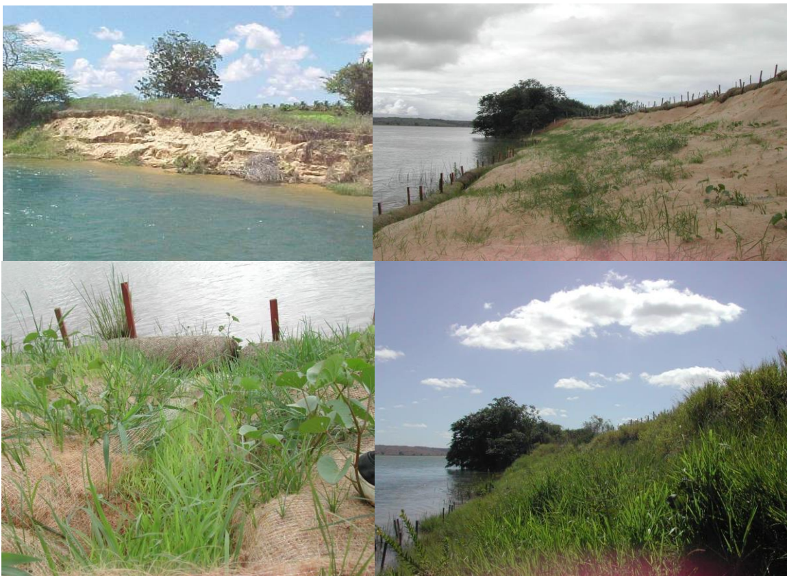
Figure 6. The use of soil bioengineering techniques to control erosion (Holanda et al. , 2005).
