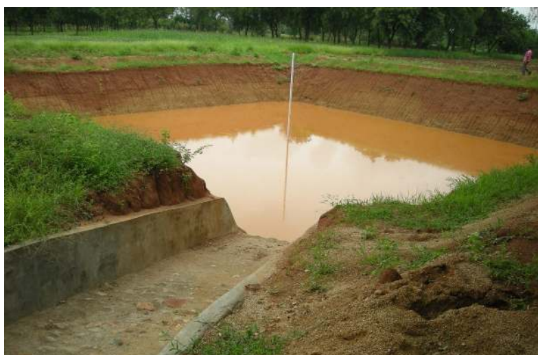
Figure 3. Farm pond for rain-water harvesting in Telengana, India.
