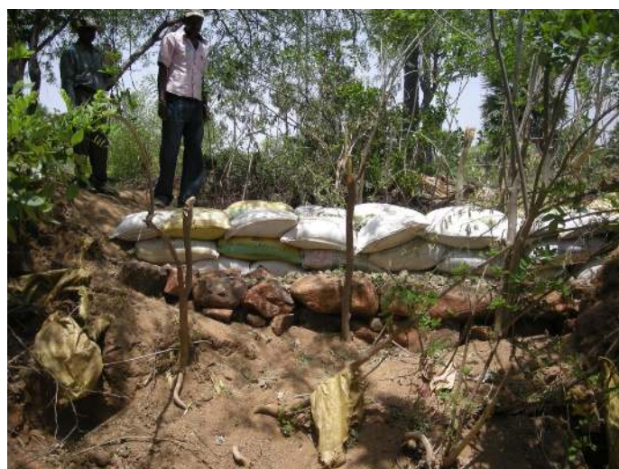
Figure 5. Sand bag structure for gully control in Telengana.
