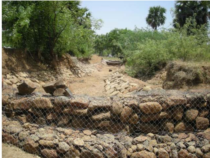
Figure 4. Stone pitching and stepped gabion for gully control in Telengana.
