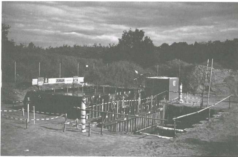
Figure 6.26 The construction excavation at the test site
