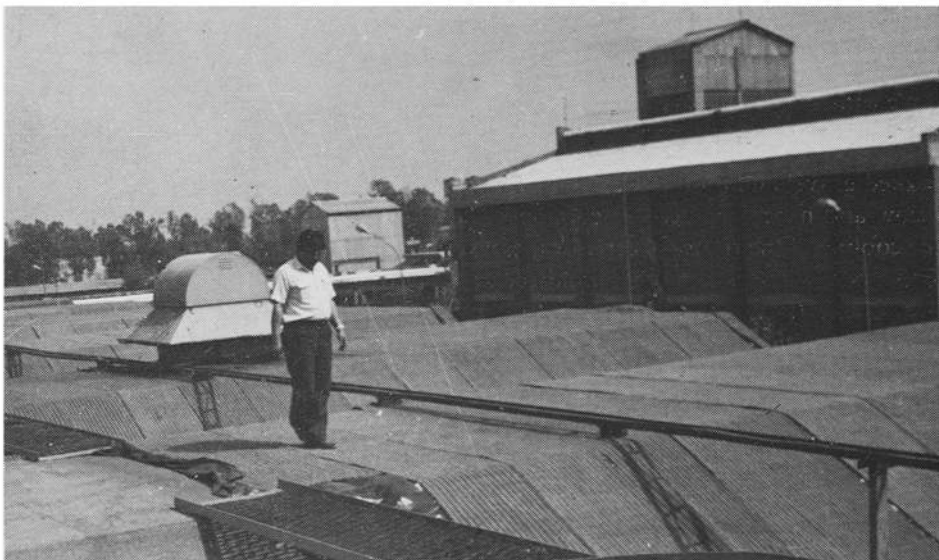
Figure 10. Roof fabric system at Modipuram – laying of coir matting.
