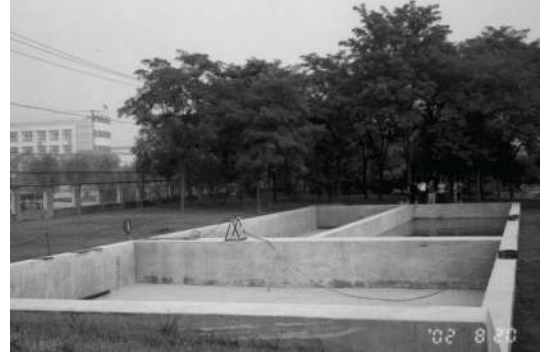
FIGURE 6: Photo of the recharge pool.
