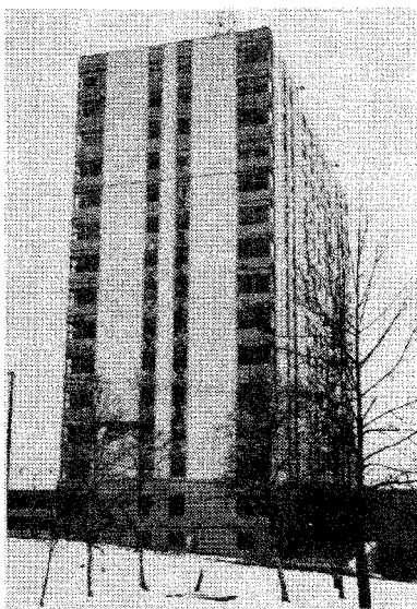
Fig. 13 A 14 storey building in Anchorage during the March 27, 1964 Alaska earthquake 17.
