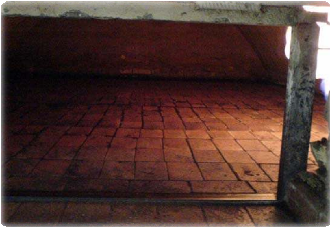
Figure 3. Interior of a Barbari oven, which is covered with Russian bricks.
