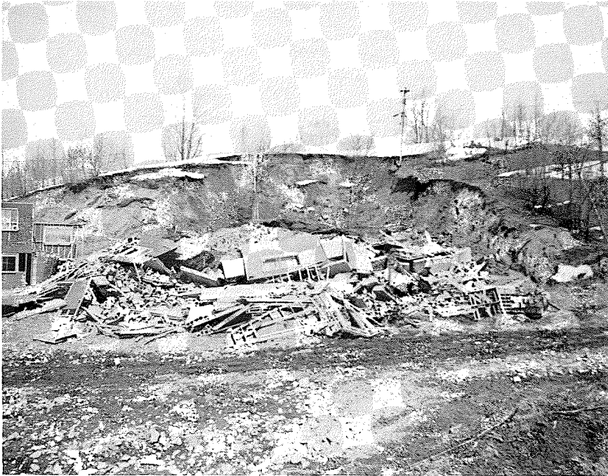
FIG. 2. Slide No. 2 and wreckage of partially completed row house.
