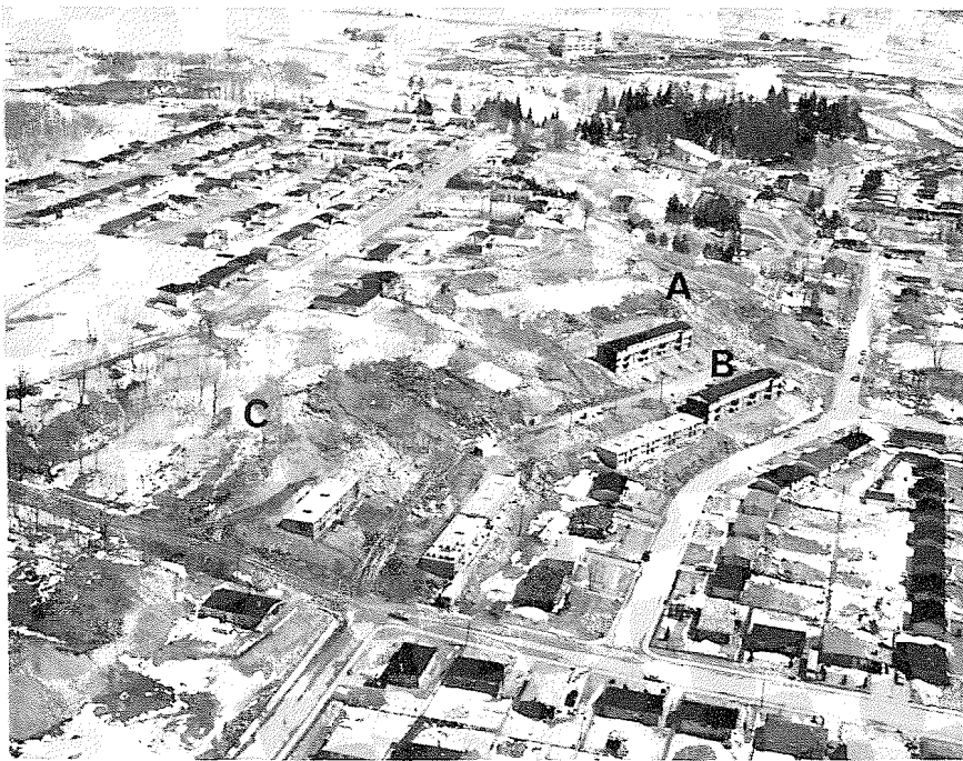
FIG. 3. Aerial view of landslide site. A. Slides 1, 3, 4, and 5. B. Le Coteau St. C. Slide 2.
