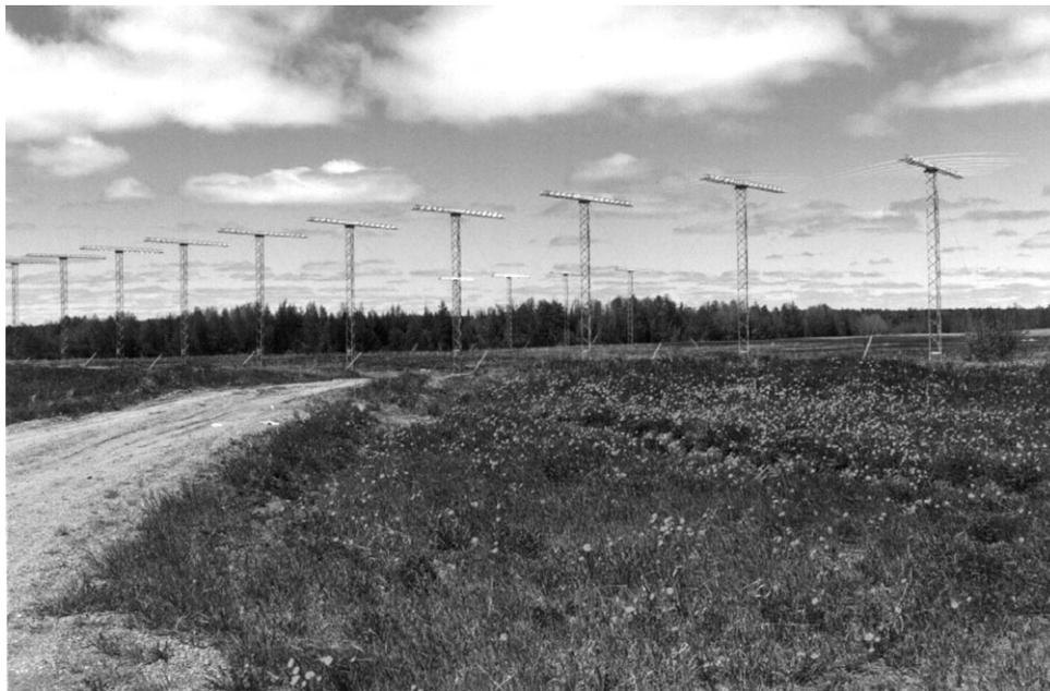
**Fig. 9.** View of antenna arrays of the SuperDARN HF radar located at Kapuskasing, Ontario.
