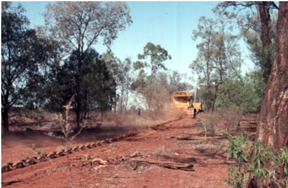
Figure 2. Clearing of aboveground biomass
