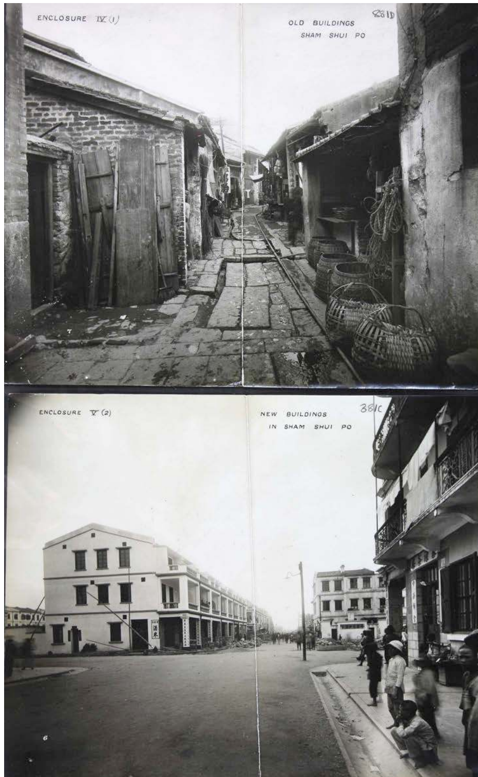
Figure 4.14. & 4.15. A comparison between “insanitary” village dwellings and the new “tenements” that replaced them, Shumshuipo, 1918. (Source: The National Archives of the U.K.: Public Records Office, London).
