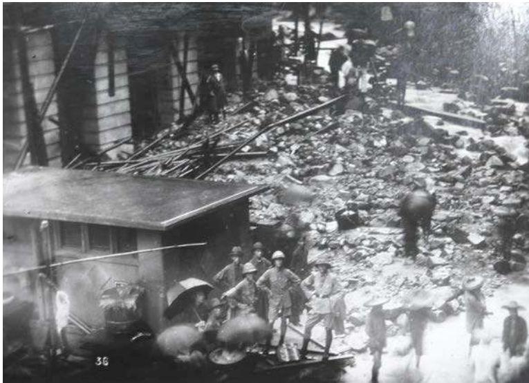
Figure 4.11. A scene of a house collapse in Victoria. (Source: The National Archives of the U.K.: Public Records Office, London).
