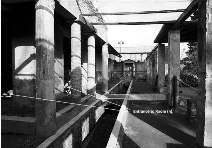
Fig. 9.2 Pompeii, Casa di Octavius Quartio (II 2,2). Euriptus area with entrances to Room (h).
