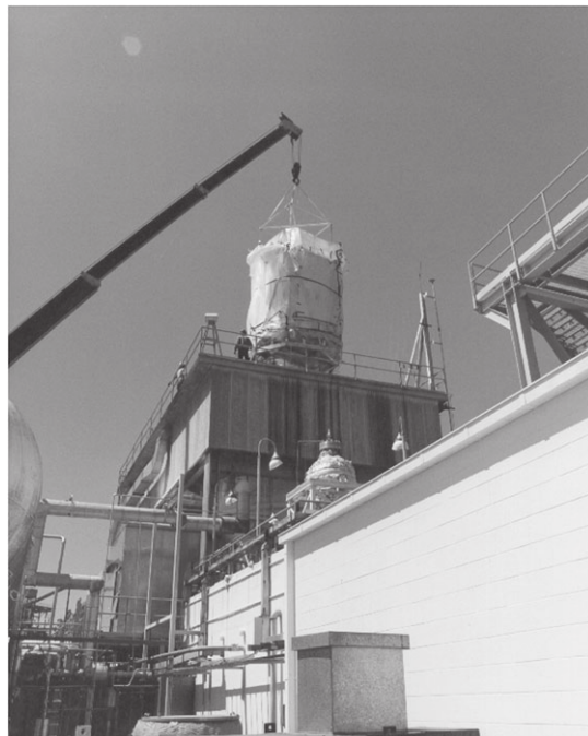
Figure 46. MHTB installation in test stand 300 vacuum chamber.
