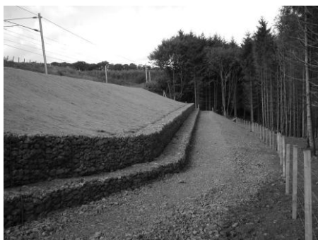
(e) Upgraded embankment slope.
