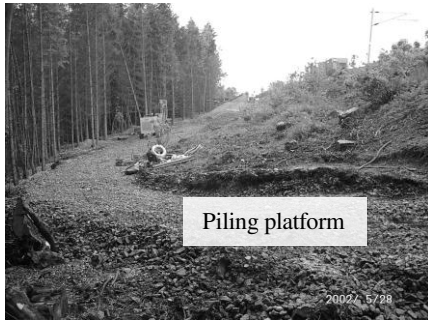
(a) Haul road to piling platform.
