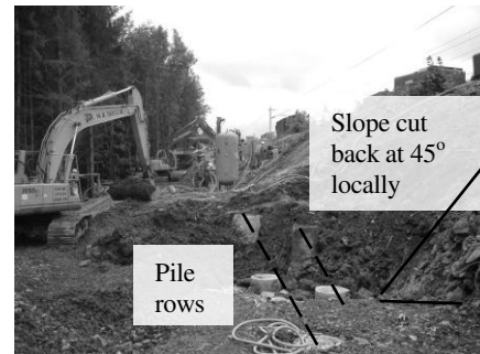
(b) Piling works.
