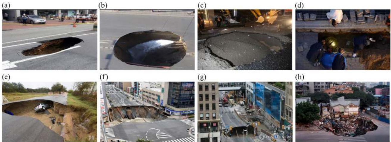
Figure 1. Ground subsidence near subways: (a) Seokchon subway station, (b) Bakchon subway station, (c) Samseongjungang subway station, (d) Janghanpyeong subway station in South Korea, (e) Texas in the US, (f) Fukuoka in Japan, (g) Ottawa in Canada and (h) Guangzhou in China.
