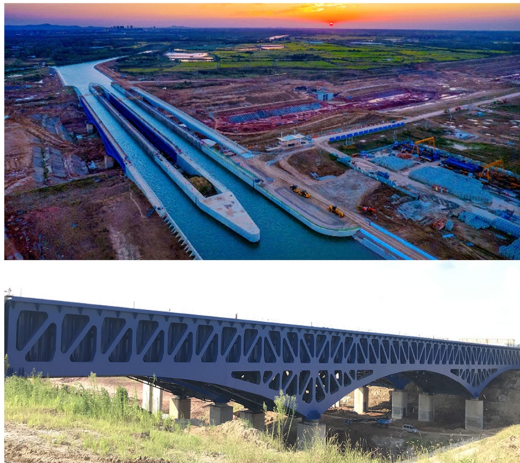
Fig. 5 The world's longest-span navigable aqueduct bridge: the Pi River Bridge
