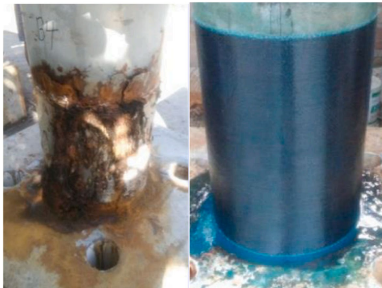
Fig. 15 The plastic hinge area of bridge pier is modified with CFRP
