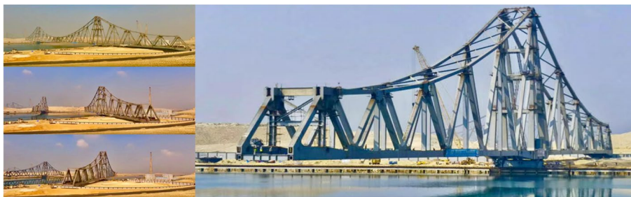
Fig. 6 The New El Felden Railway Open Bridge in Egypt
