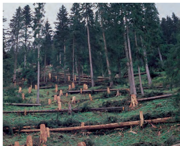
Fig 9 Rockfall protection by obstacles consisting of logs positioned on the slope (Photo: Bernhard Maier).
