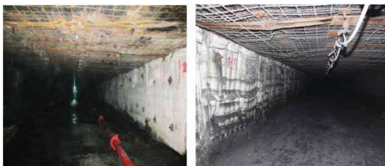
Figure 13—Pumpable concrete wall in GERT (Cui, 2014)
