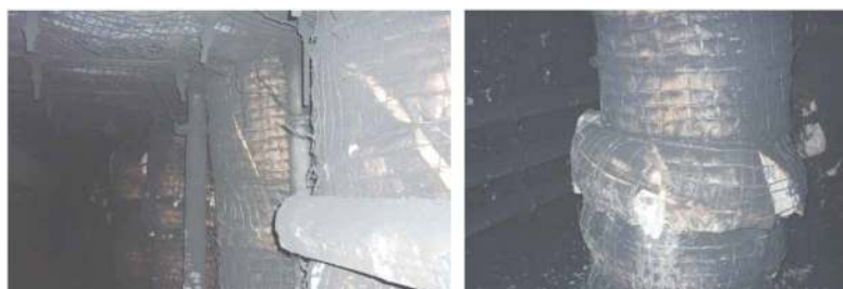
Figure 18—GERT with HWM-filled plastic bag column (Yu et al. , 2019)
