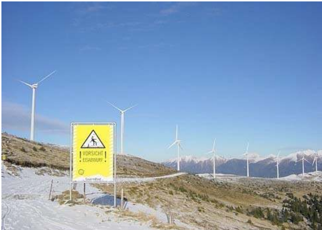
Figure 9. Warning against shedding ice fragments at Tauernwindpark in Austria. Photo from http://www.tauernwind.com .
