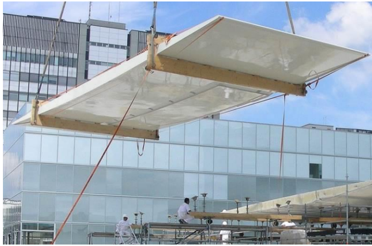
Fig. 8. Lightweight GFRP sandwich roof (Keller et al., 2008)
