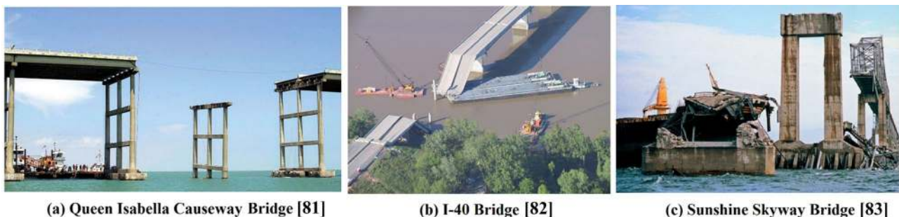
Fig. 13 The collapse of several bridges in the USA due to vessel collisions
