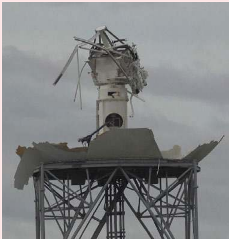
Fig. SB4.2. Heavily damaged National Weather Service Lake Charles radar following Hurricane Laura. (Image courtesy of Brett Adair, Live Storms Media.)
