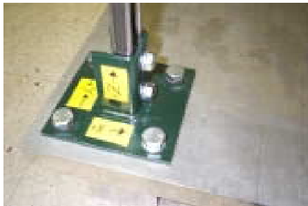
Figure 8: the connection to the base plate
