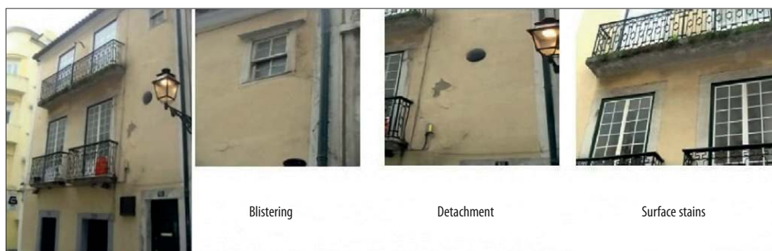
Fig. 2. Case study representative of the end of the service life of façade paintings (degradation severity around 20%)
