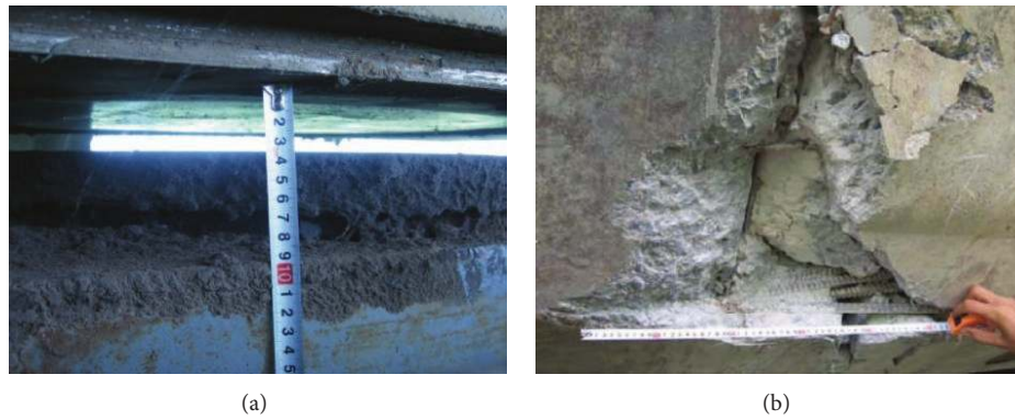
FIGURE 2: (a) Auxiliary pier detachment and (b) damage situation of segment Tianjin direction.
