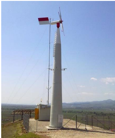
FIGURE 22. Wind turbine photo. SIHDC is installed inside the metallic container located behind the tower.
