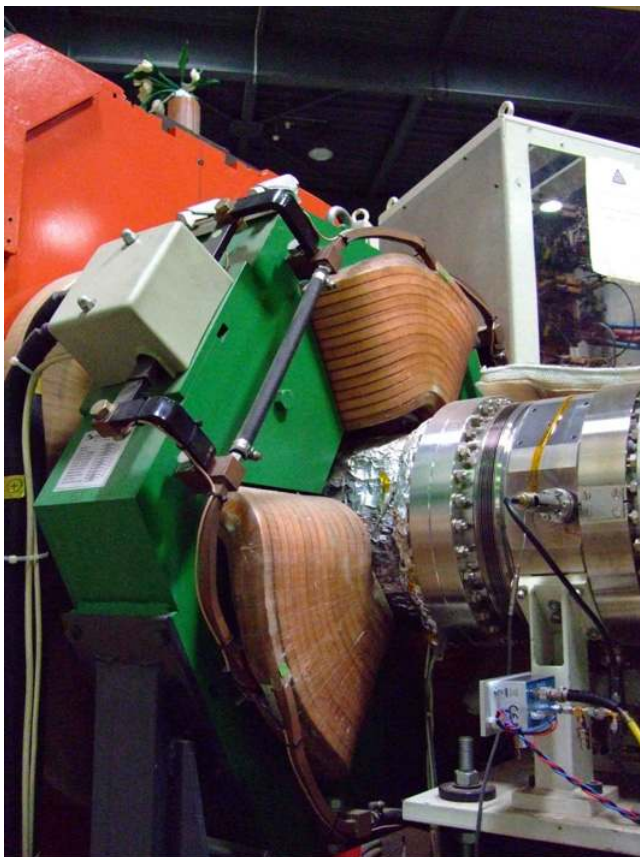
Fig. 32. TSR sextupole magnet. In the front of the sextupole magnet a capacitive pick up to measure the closed orbit of the ion beam is recognizable.
