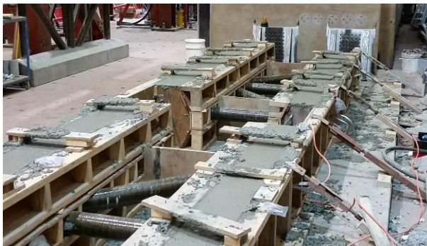
(c) Top and Bottom Chords after Casting
