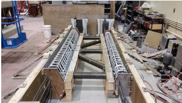
(a) Top and Bottom Chords before Casting
