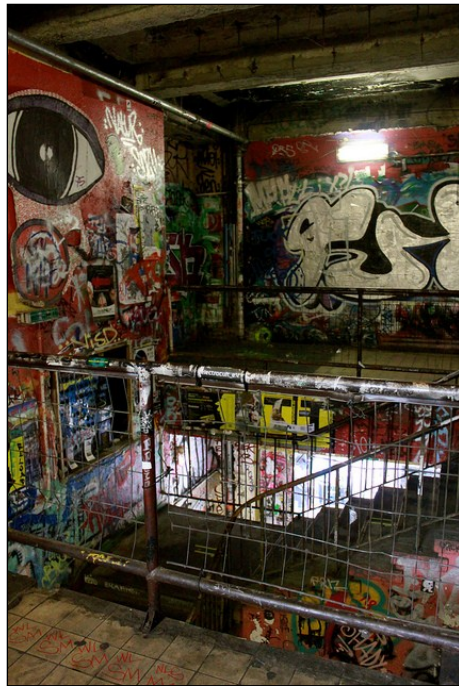
Figure 30 Tacheles Main Stairwell
