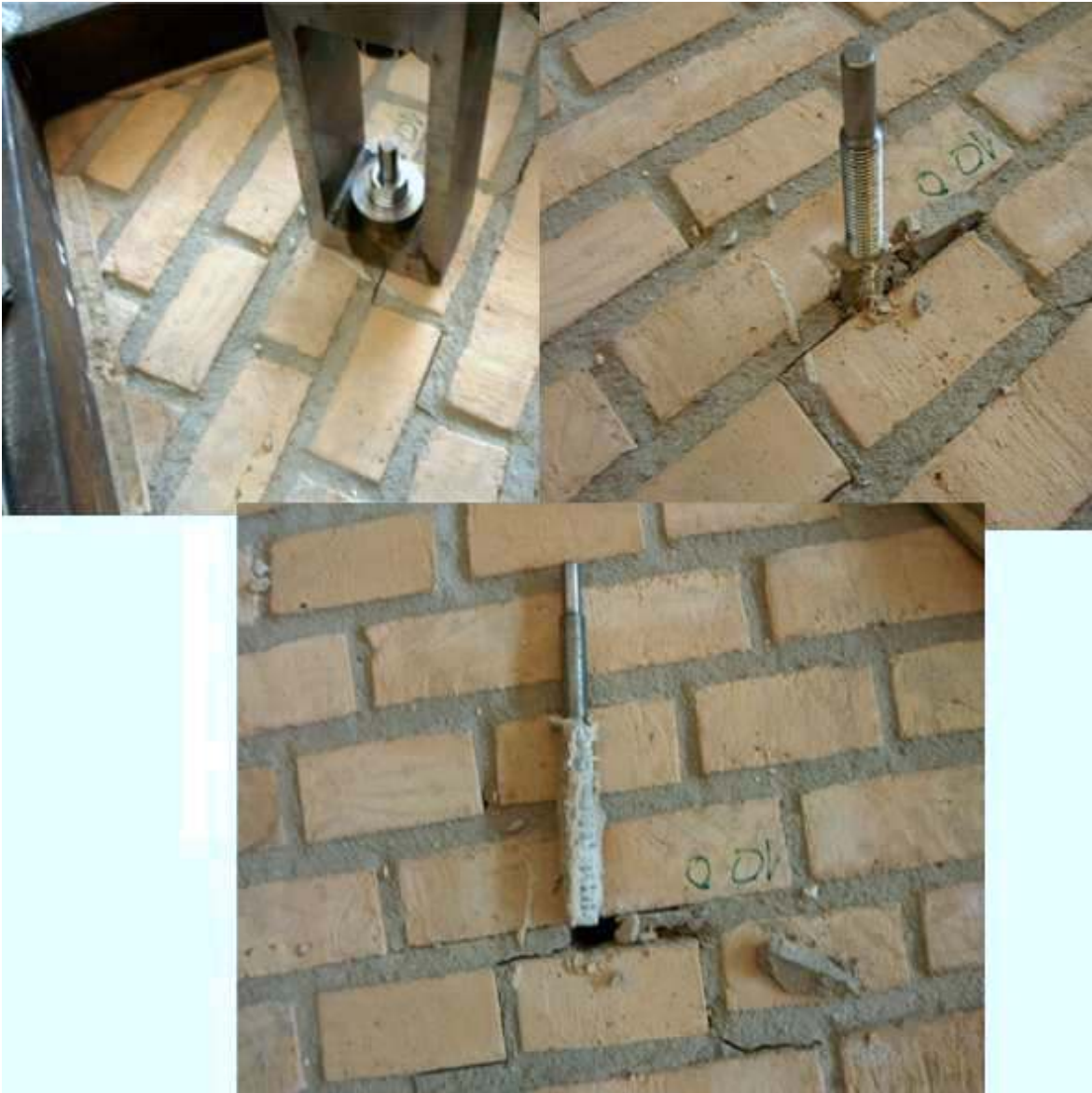
Figure A.101: The failure mode observed
