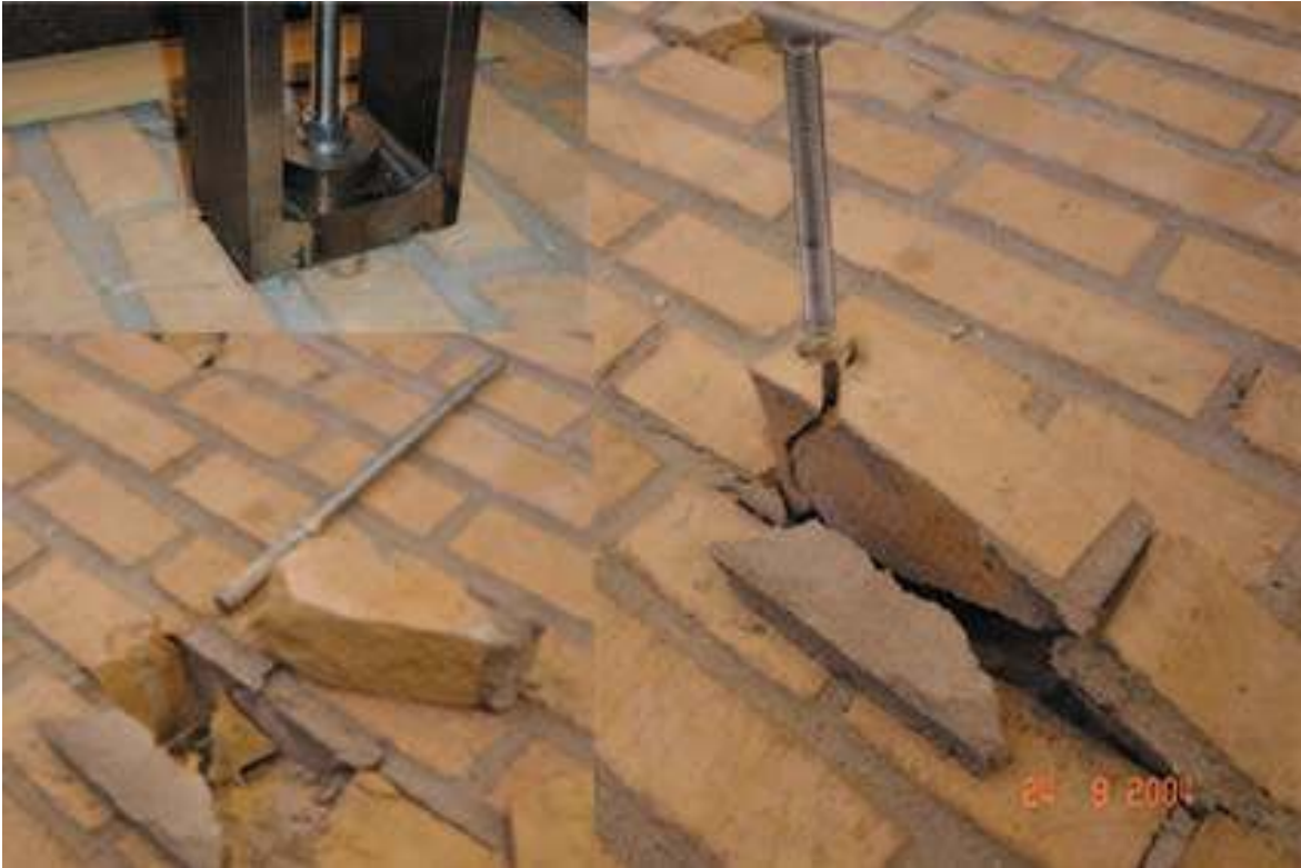
Figure A.3: The failure mode observed
