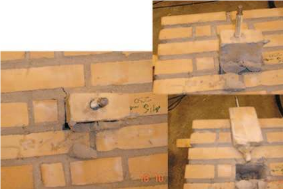
Figure A.125: The failure mode observed
