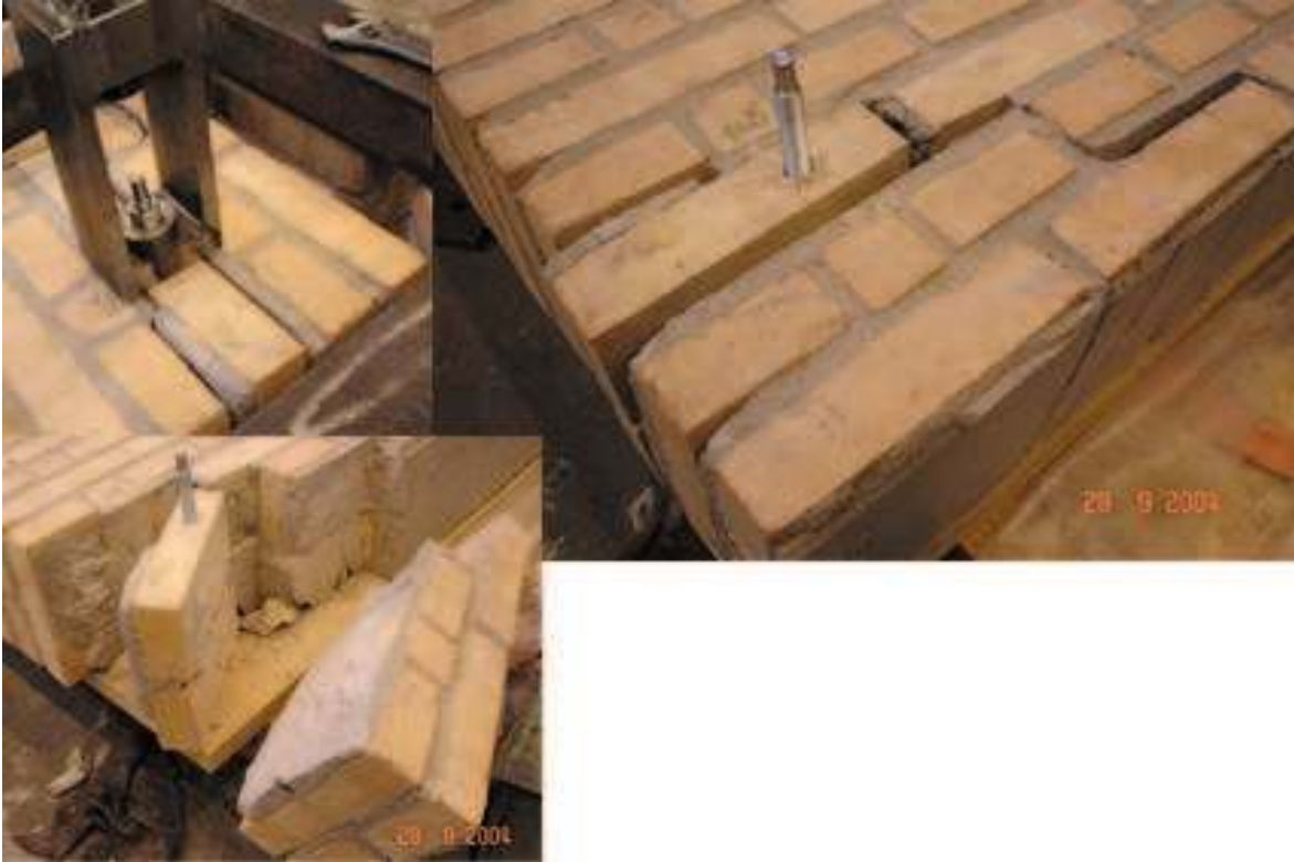
Figure A.119: The failure mode observed
