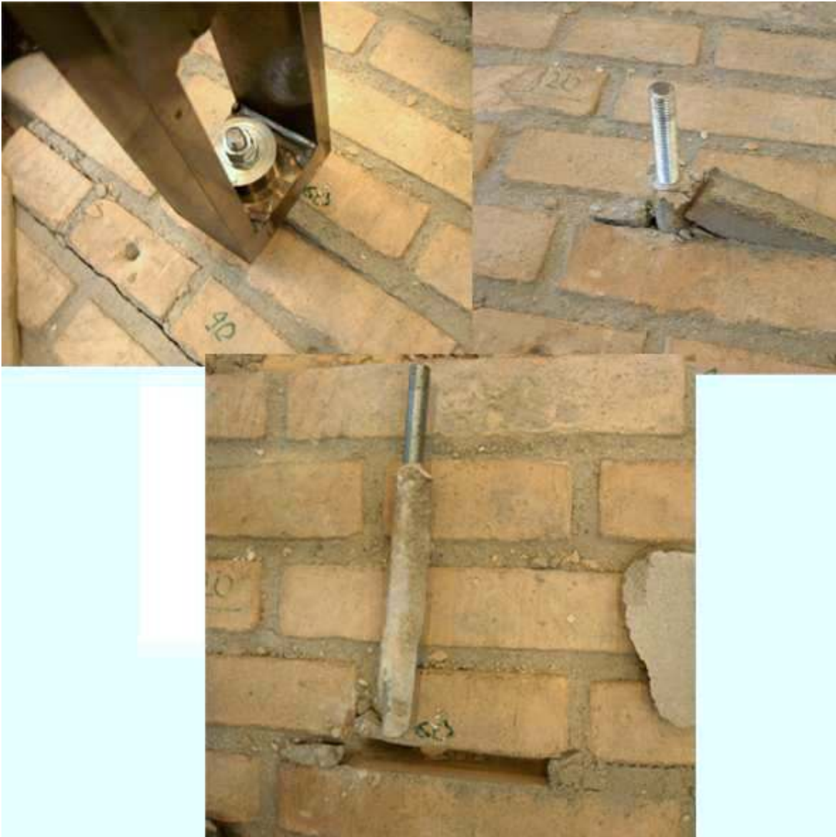
Figure A.99: The failure mode observed
