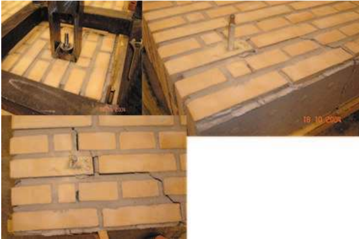
Figure A.121: The failure mode observed
