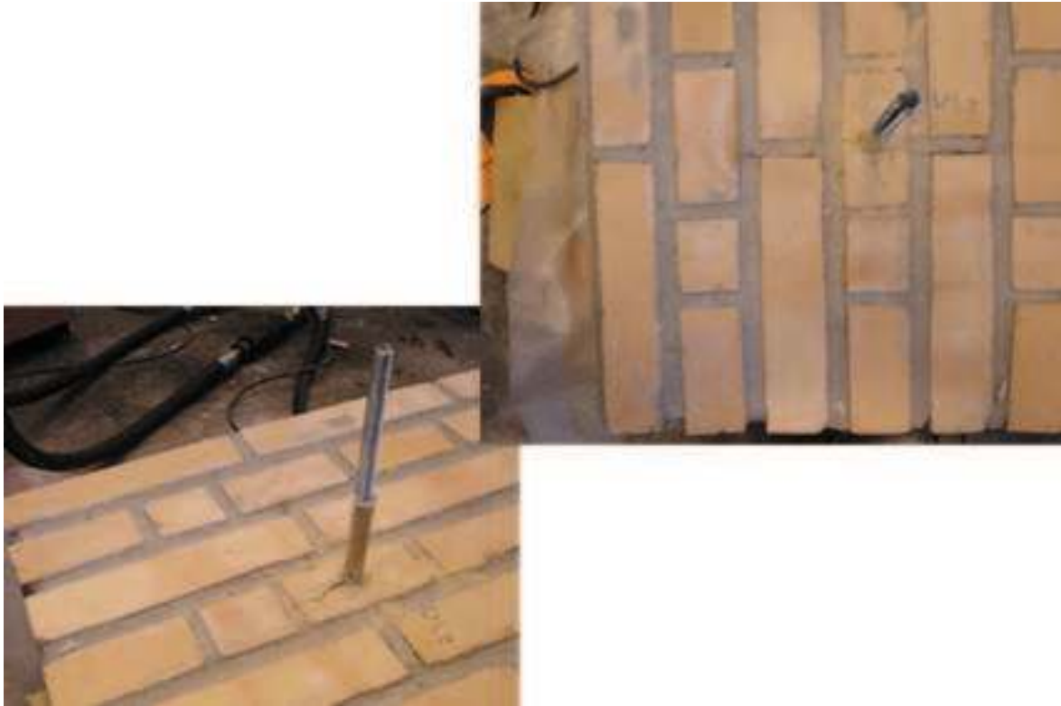
Figure A.113: The failure mode observed
