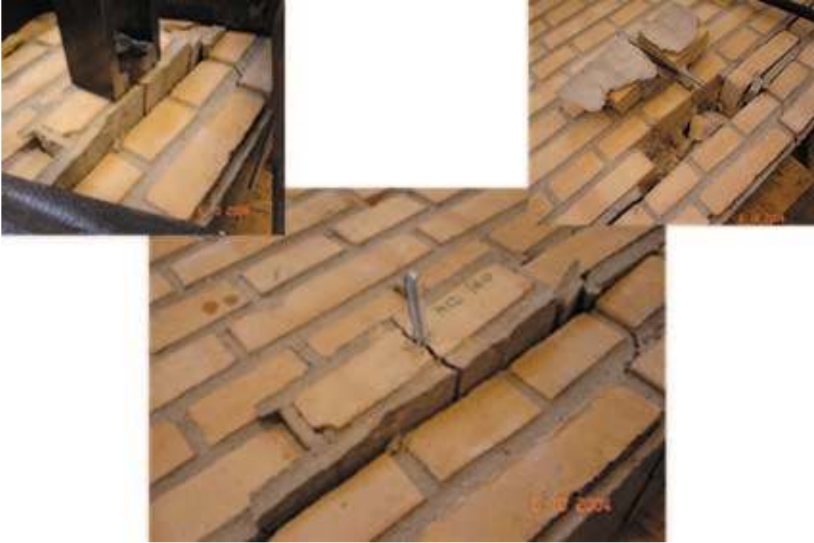
Figure A.141: The failure mode observed
