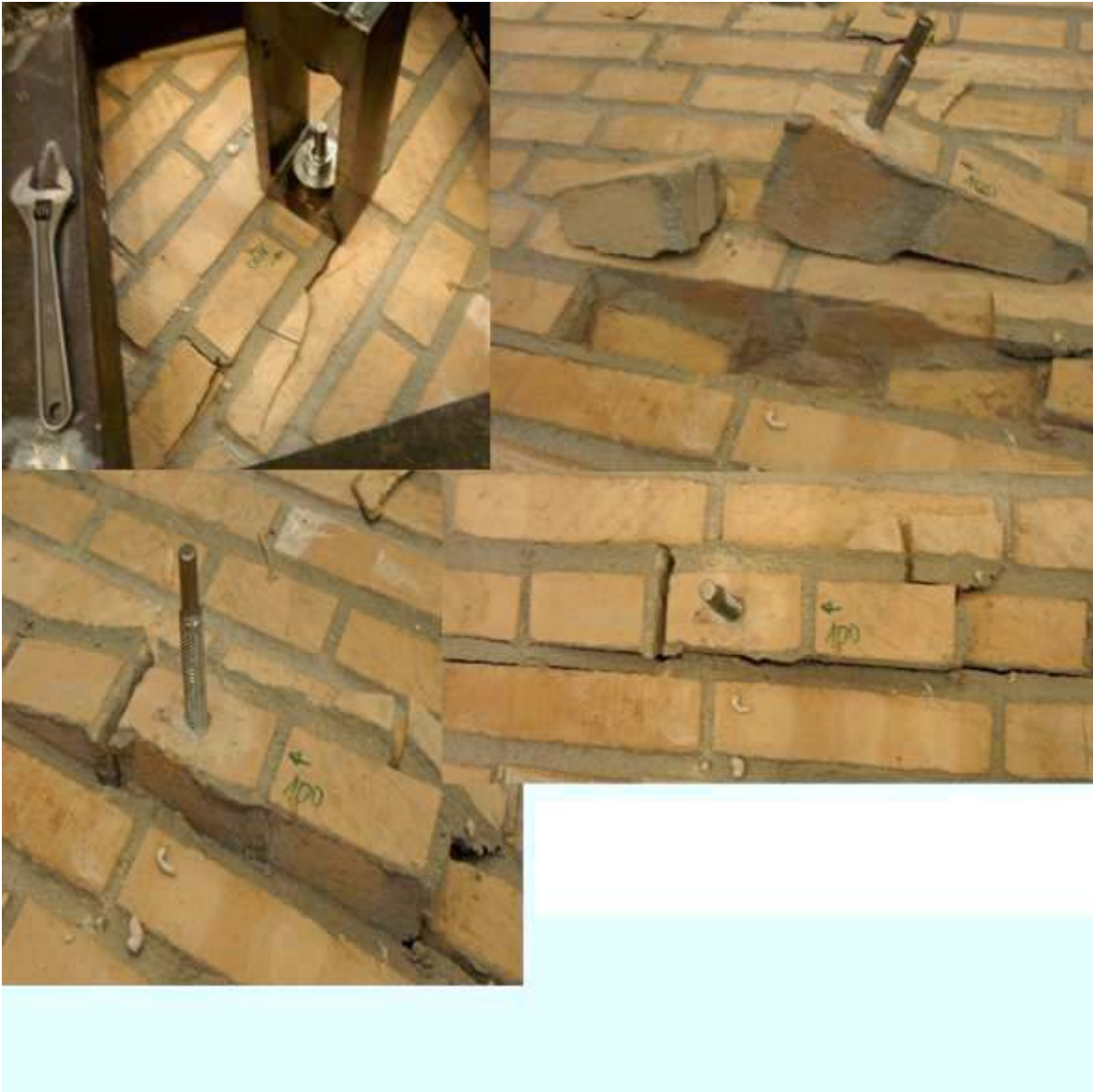
Figure A.77: The failure mode observed
