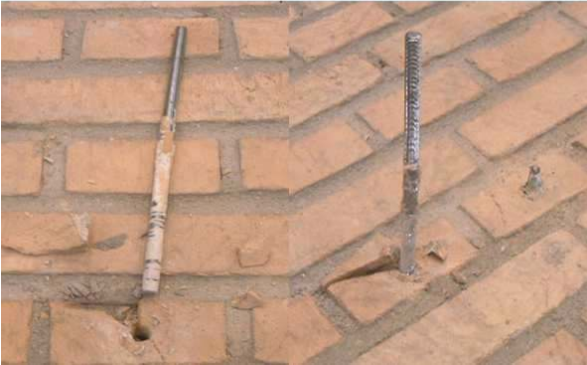
Figure A.65: The failure mode observed
