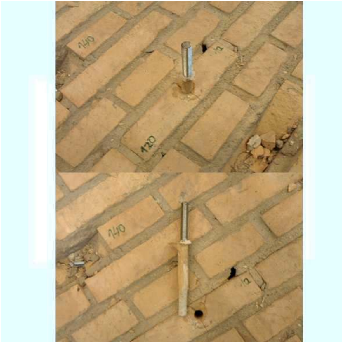
Figure A.25: The failure mode observed
