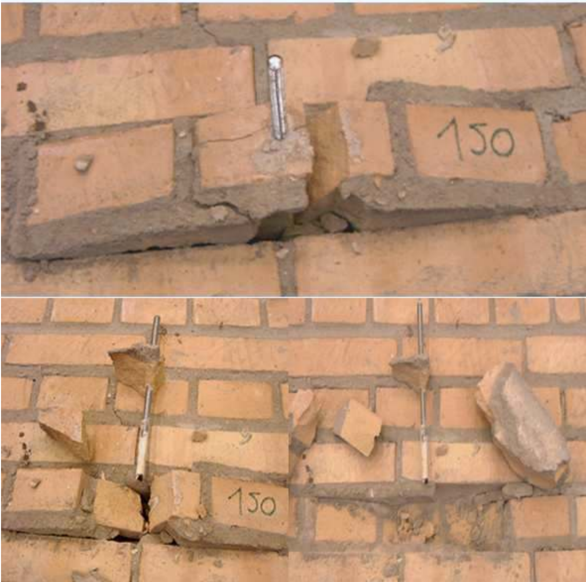
Figure A.63: The failure mode observed
