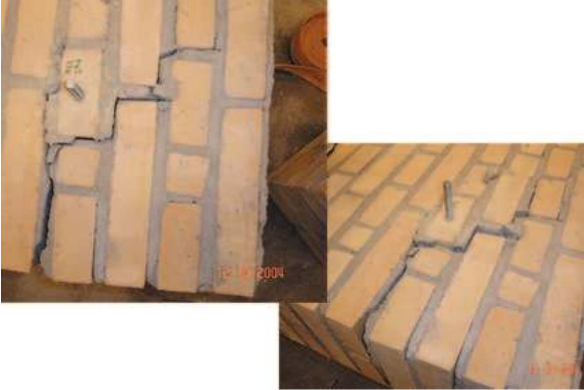
Figure A.115: The failure mode observed
