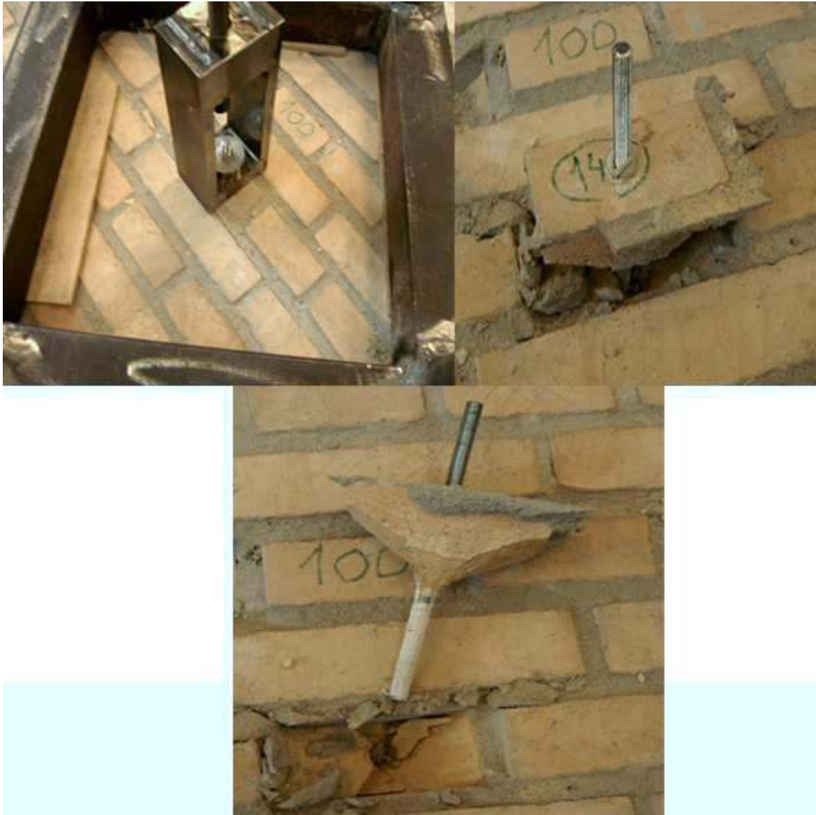
Figure A.61: The failure mode observed
