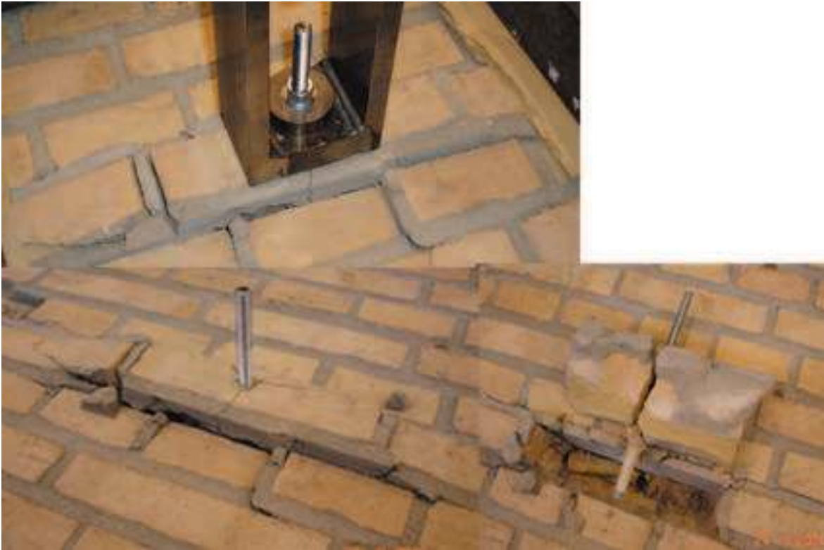
Figure A.7: The failure mode observed
