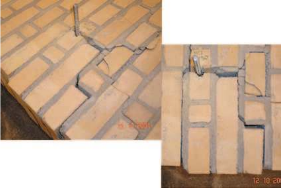
Figure A.131: The failure mode observed
