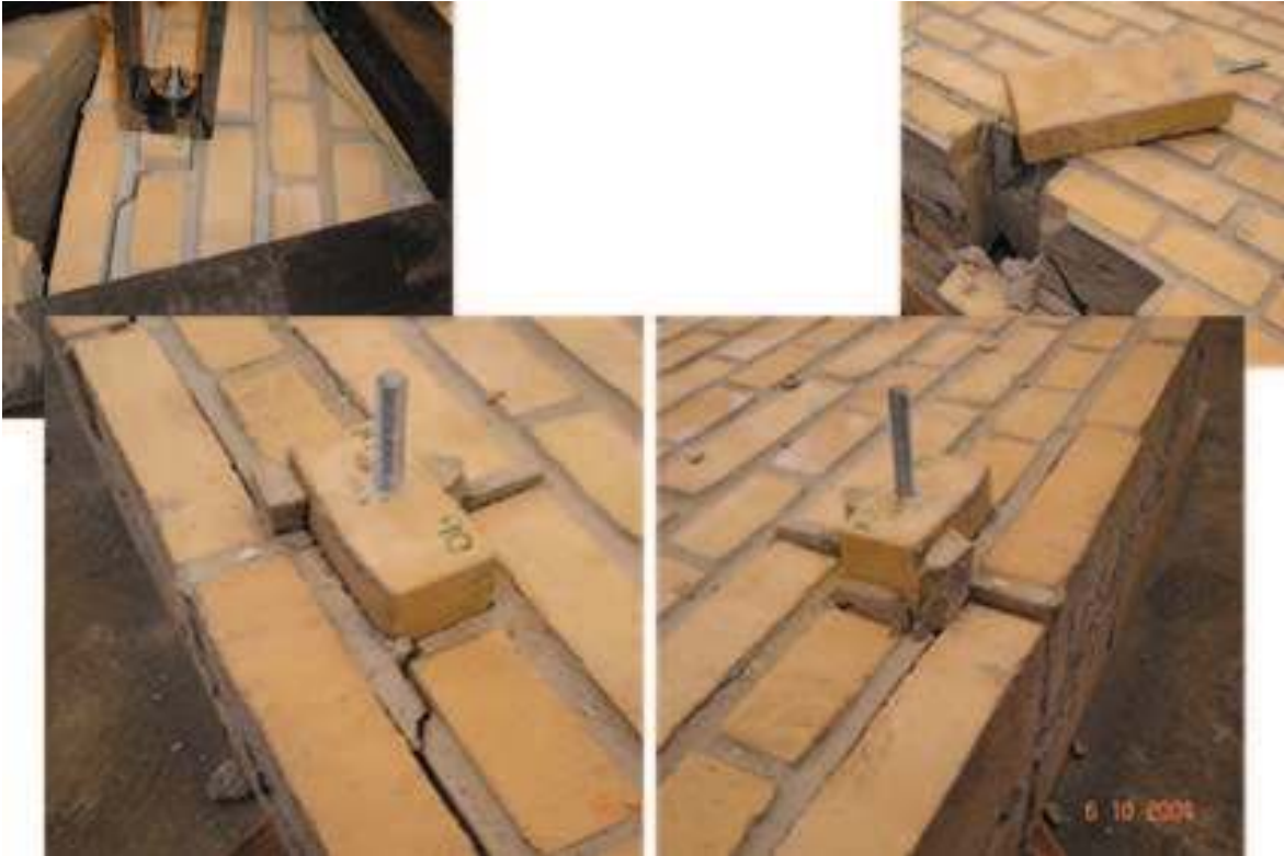
Figure A.139: The failure mode observed
