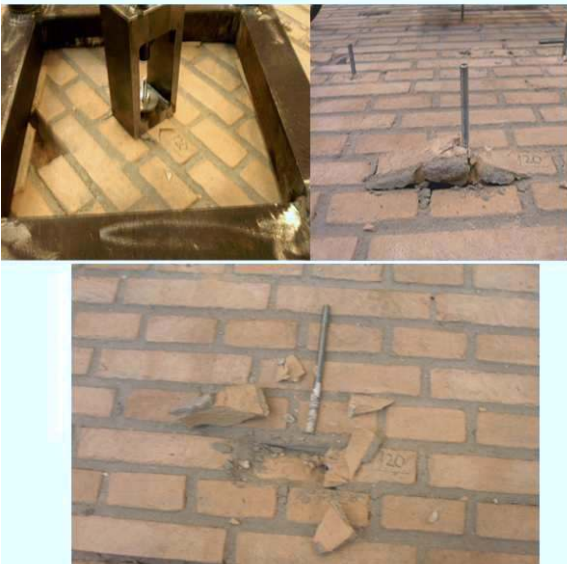
Figure A.17: The failure mode observed
