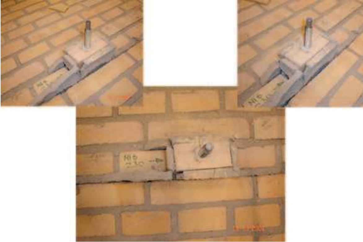
Figure A.149: The failure mode observed
