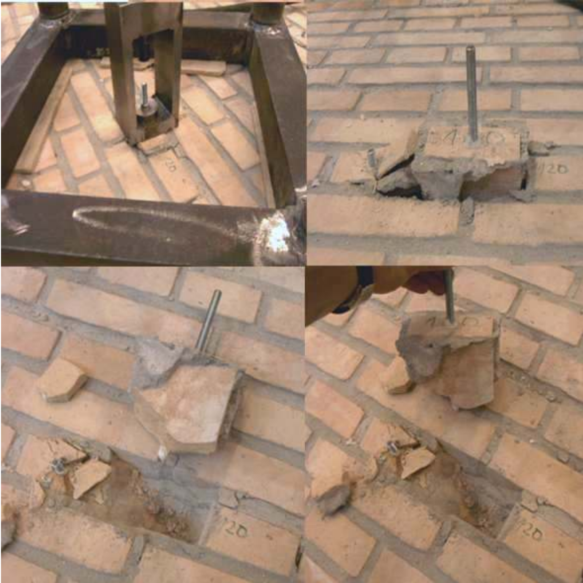
Figure A.57: The failure mode observed
