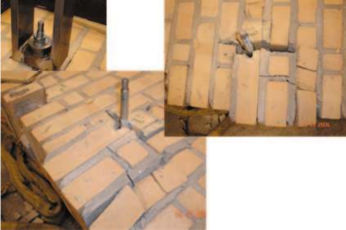
Figure A.135: The failure mode observed
