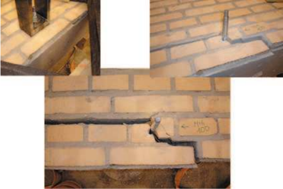
Figure A.145: The failure mode observed
