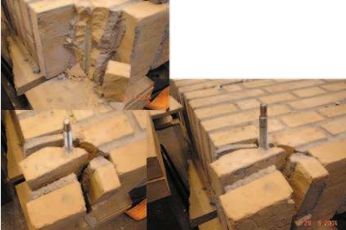
Figure A.117: The failure mode observed
