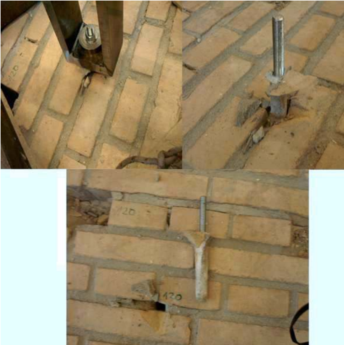
Figure A.95: The failure mode observed
