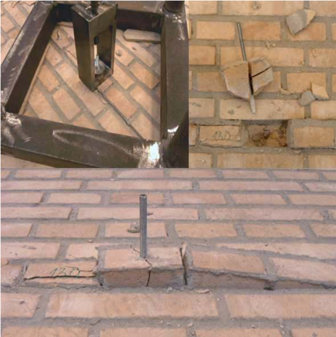
Figure A.59: The failure mode observed
