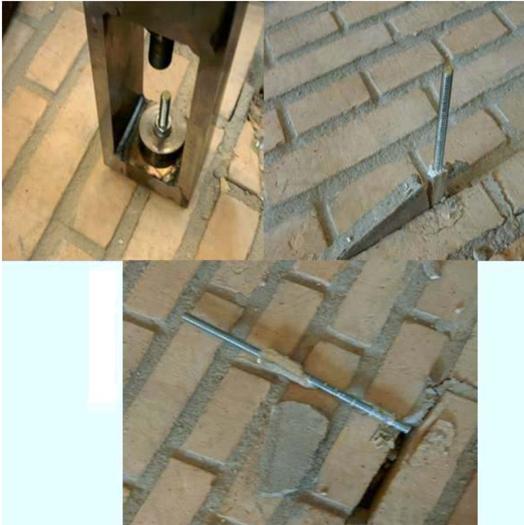
Figure A.91: The failure mode observed
