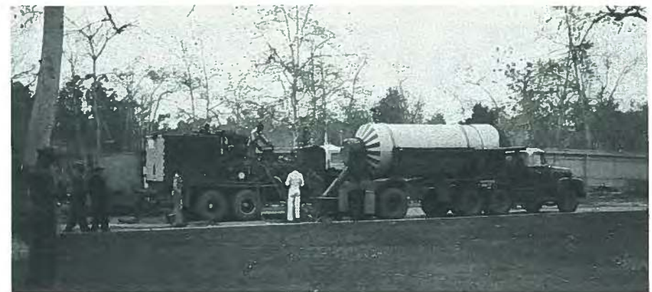
Fig. 11. Halliburton grouting the girders.
