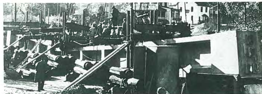
(c) Girder after failure.
