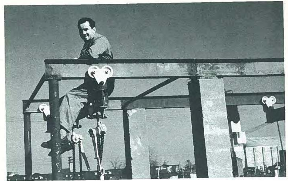
Fig. 21. Jean Muller, a welcome visitor to Prestressed Concrete of Colorado, takes a break on the support rails of the jacking assembly.
