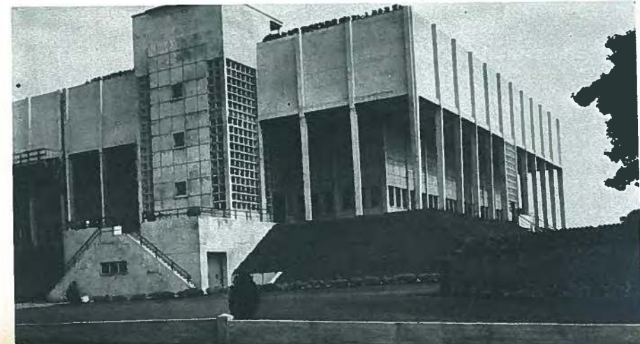
Fig. 31. Water storage reservoir and offices, Orleans, France.
