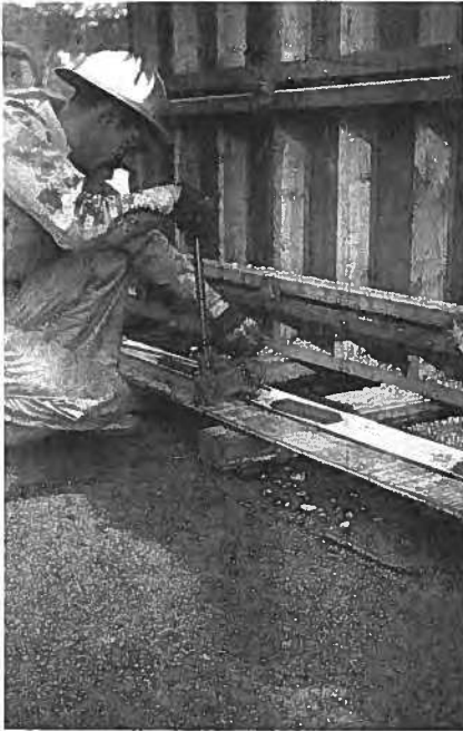
Fig. 5. Wooden trough for measuring and cutting wire.
