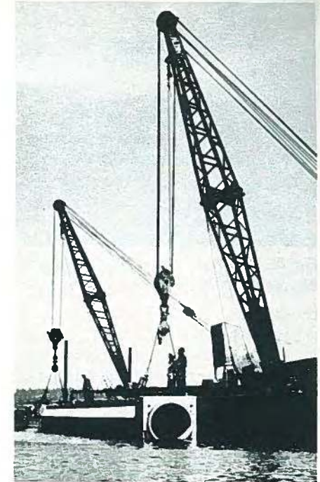
Fig. 87. 85-ton (77 t) precast prestressed hollow pipe section being installed in Lake Washington.
