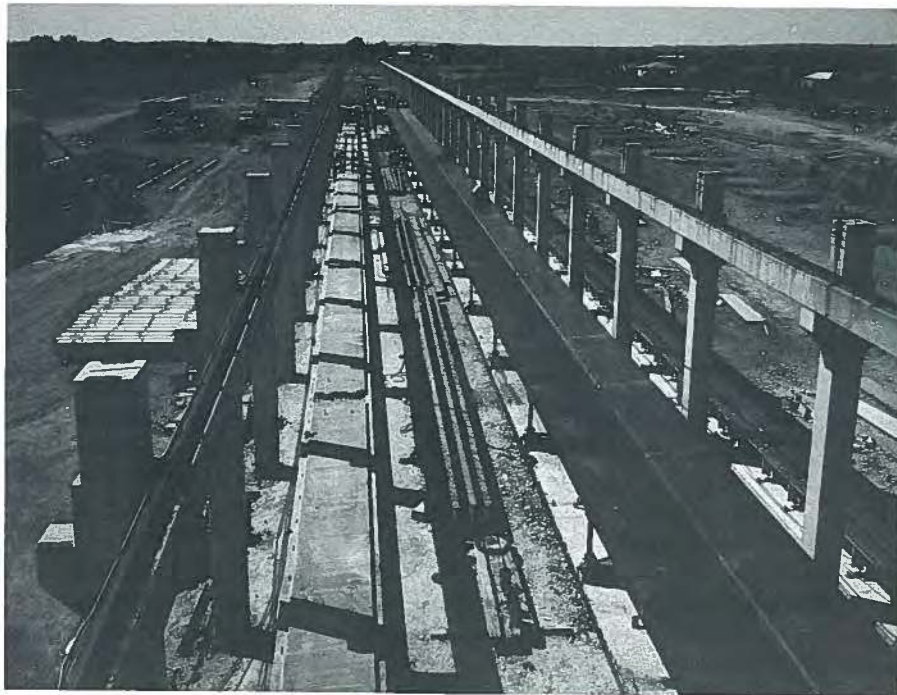
Fig. 11. The modern plant of Wilson Concrete Products under construction (1956).
