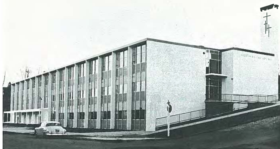
Fig. 67. Completed school, after only 6 months of construction.
