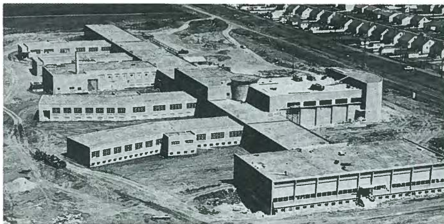
Fig. 8. School for the Deaf, Edmonton, Alberta, 1955—complete precast column and beam framing and prestressed double tee floor and roof slabs.
