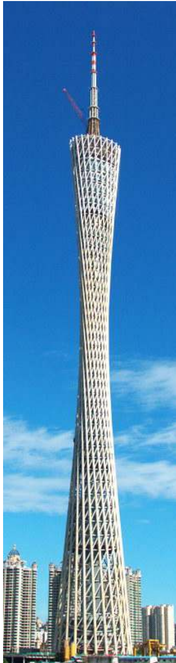
Fig. 1. Perspective view of Guangzhou New TV Tower in July 2009
