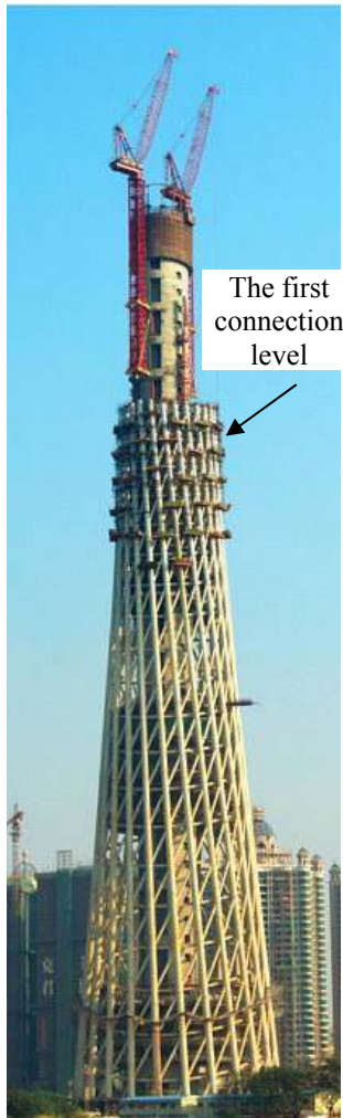
Fig. 8a. One of the critical stages of construction
