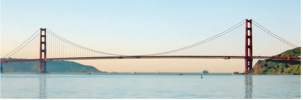
Fig. 4 The shape of the main cables of the Golden Gate Bridge is very close to a parabola. Photo courtesy of Patricia A. Browne.
