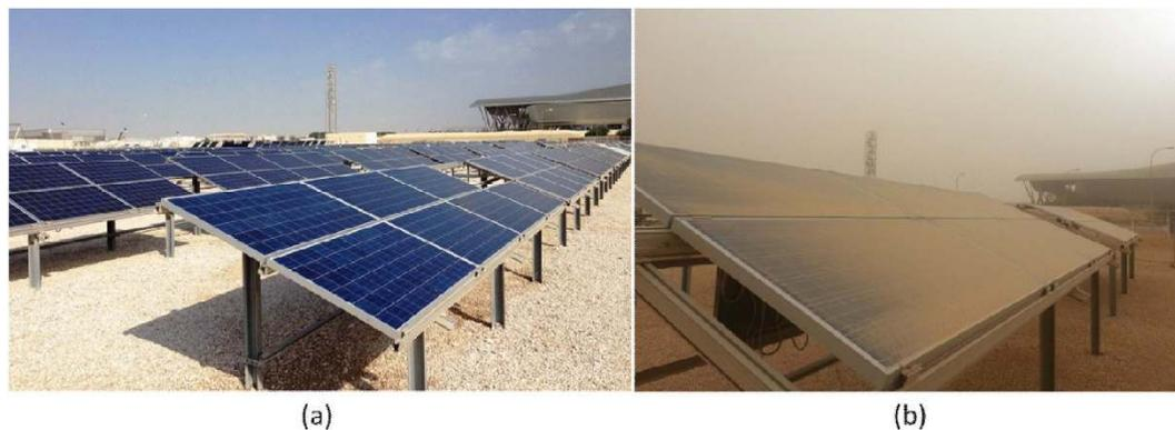
**Figure 1.** The Solar Test Facility located at the Science and Technology Park, in Doha (State of Qatar) with different PV technologies installed to study the performance and reliability of PV in Qatar climatic conditions; (a) PV modules after scheduled cleaning and (b) PV modules after dust storm inducing soiling.
